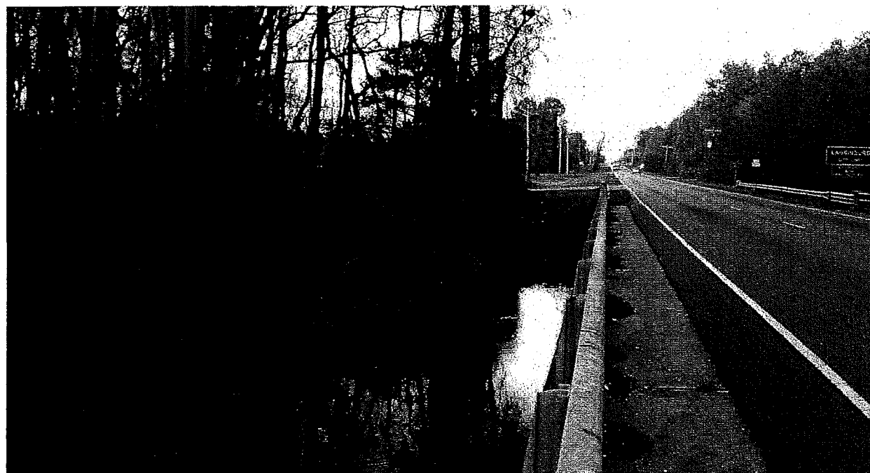
PHOTO TAKEN FROM EXISTING BRIDGE DECK FACING UP STATION TOWARD DETOUR BRIDGE END BENT 2
