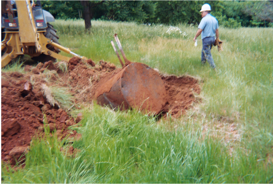
Photograph 1: Removing overburden from tank.
