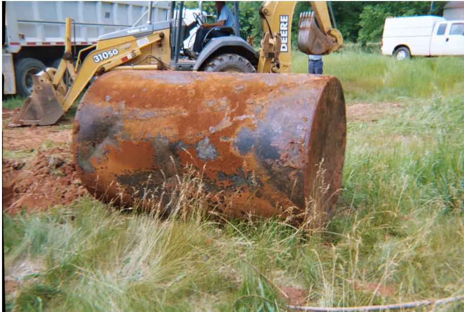
Photograph 3: Tank inspection revealed no holes or cracks.
