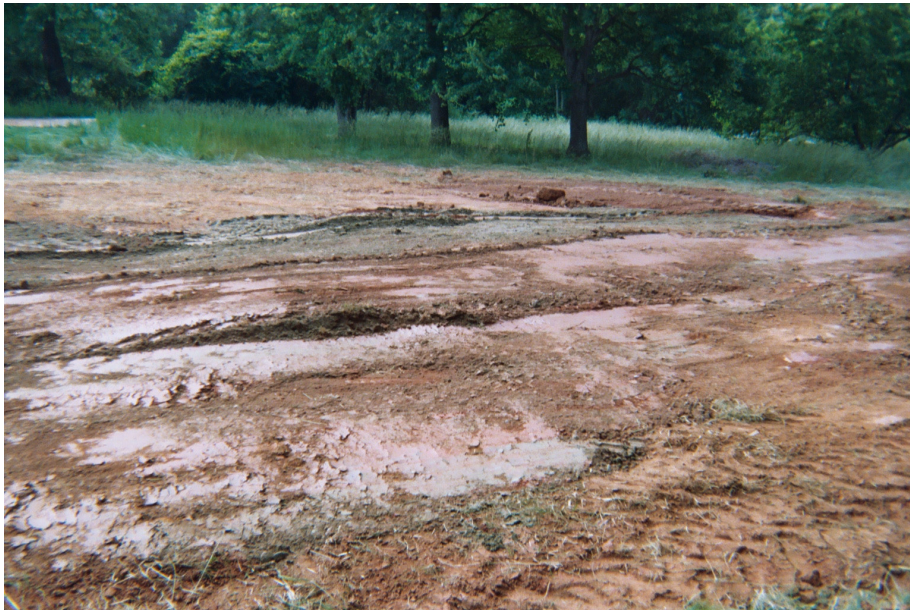
Photograph 4: Backfilling of excavation is complete.
