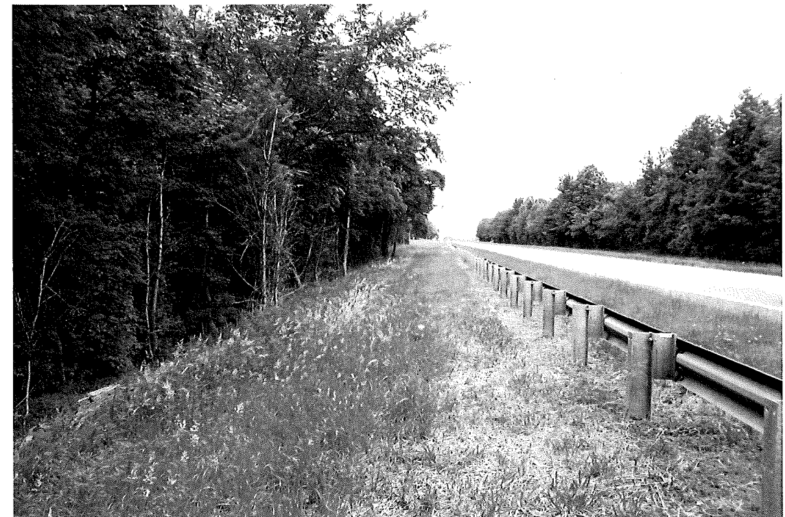
Looking right along End Bent 2 from EB2-A
