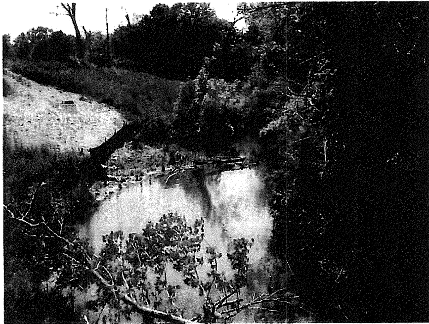
Photograph No. 8: This photograph was taken from the existing bridge, looking west (upstream).
