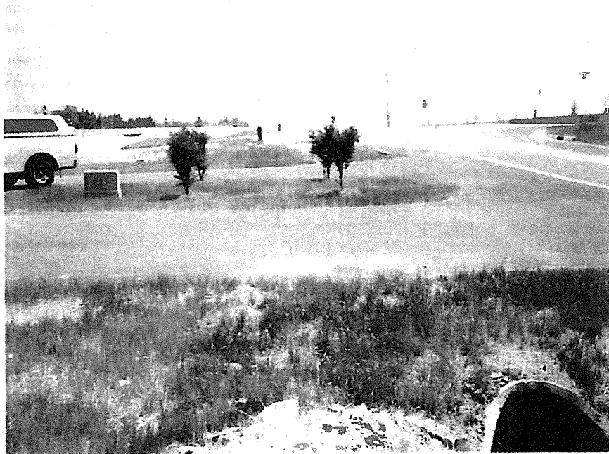
Photograph No. 2: This photograph was taken from the right side of the -L- alignment, looking south, along the proposed Retaining Wall.
