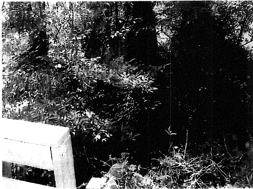
Photograph No. 10: This photograph was taken from the centerline of the -L- alignment, looking west, across proposed Interior Bent No. 2.
