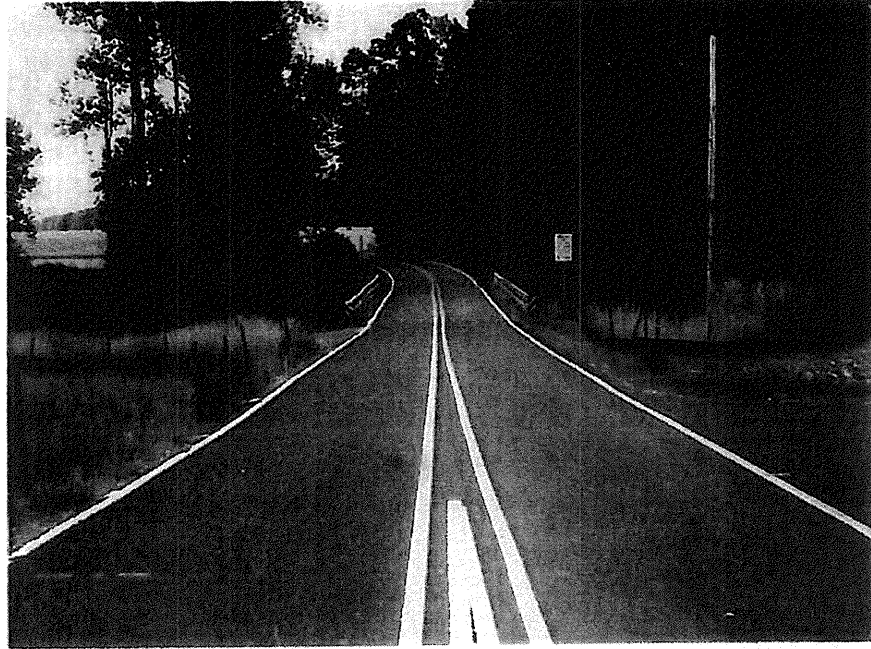
Photograph No. 3: This photograph was taken from the south approach along the centerline of the -L- alignment, looking north.
