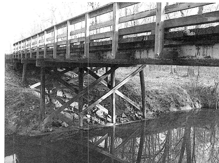
Photograph No. 4: View looking southeast at east end of bridge
