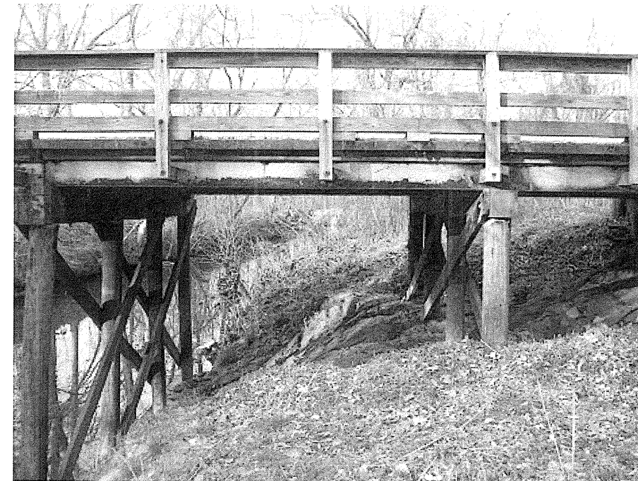
Photograph No. 3: View looking north along proposed Bent 2
