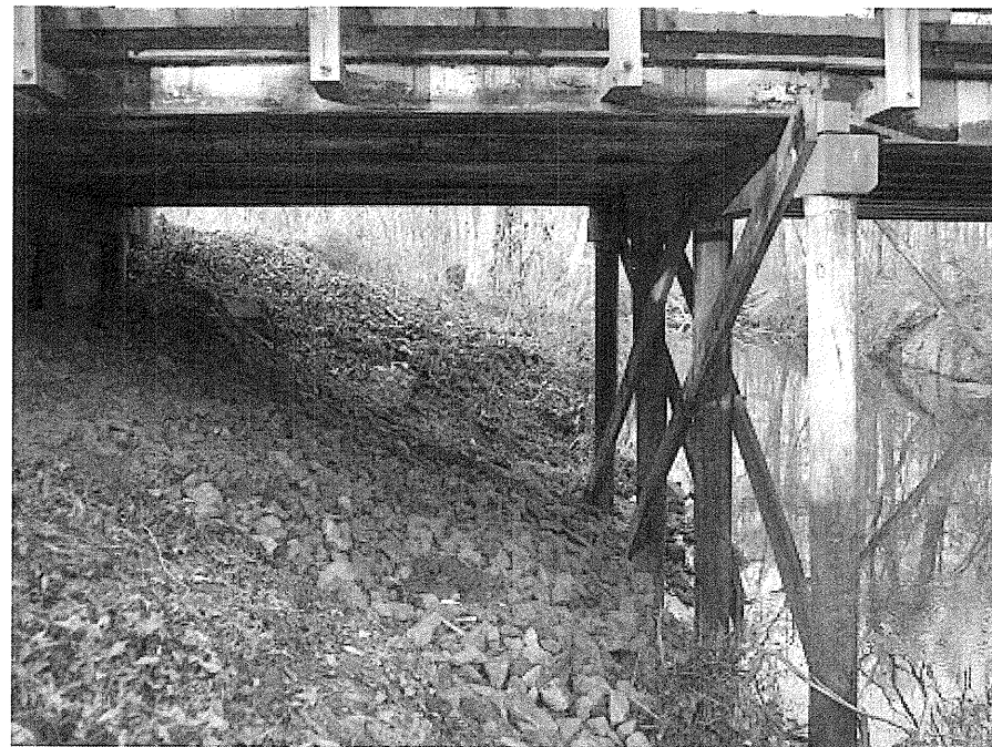
Photograph No. 2: View looking north along proposed Bent 1
