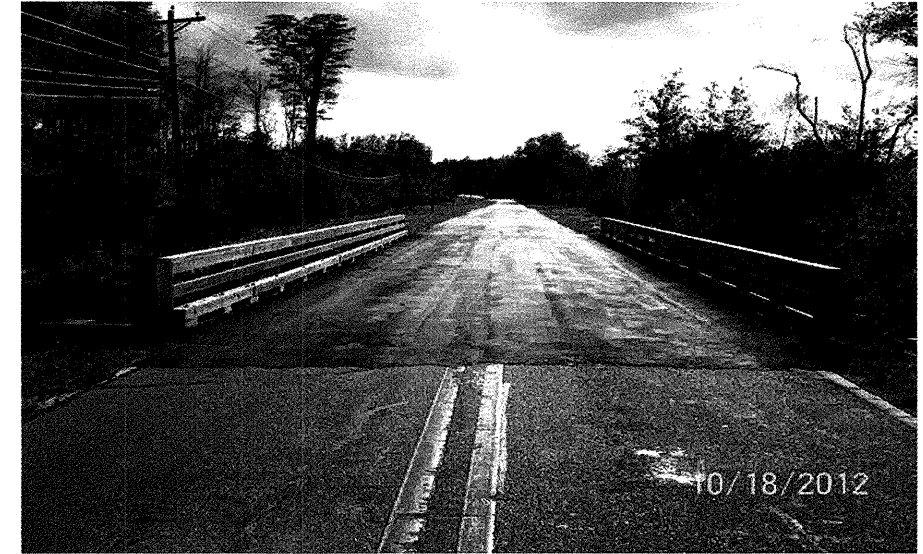
View of Bridge Looking Downstation
