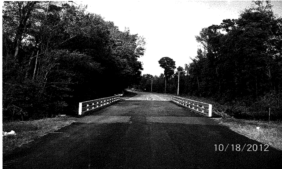
View of Bridge Looking Upstation
