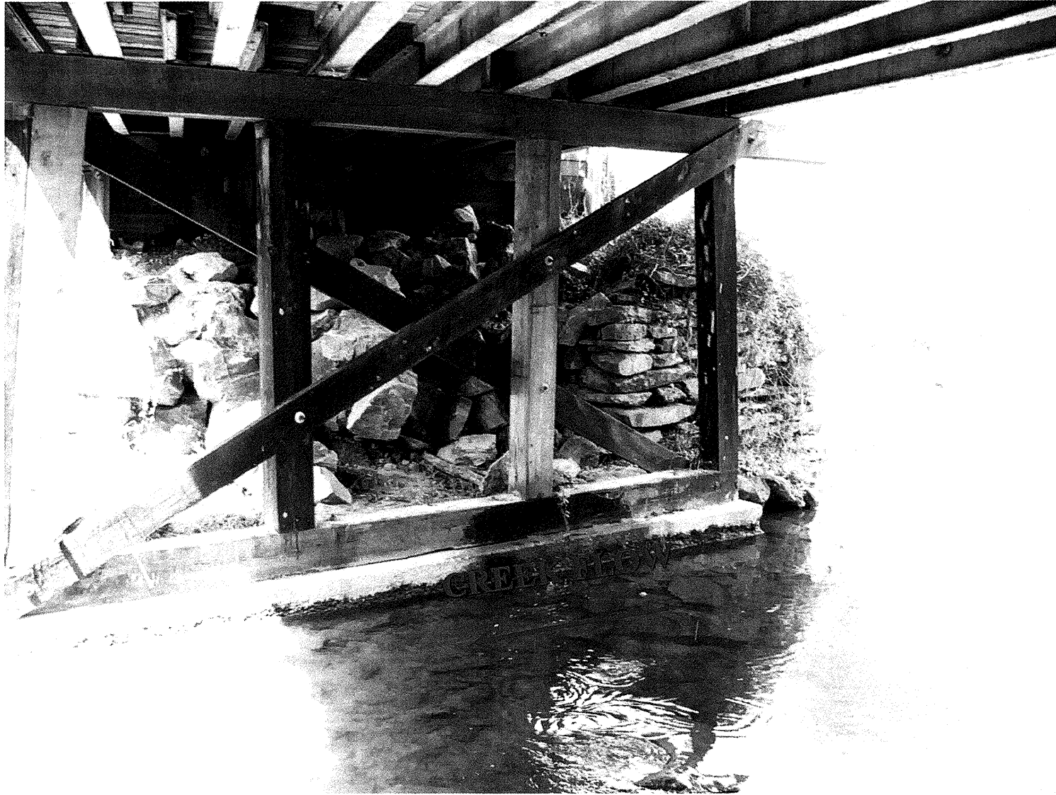
UNDER BRIDGE LOOKING WEST
