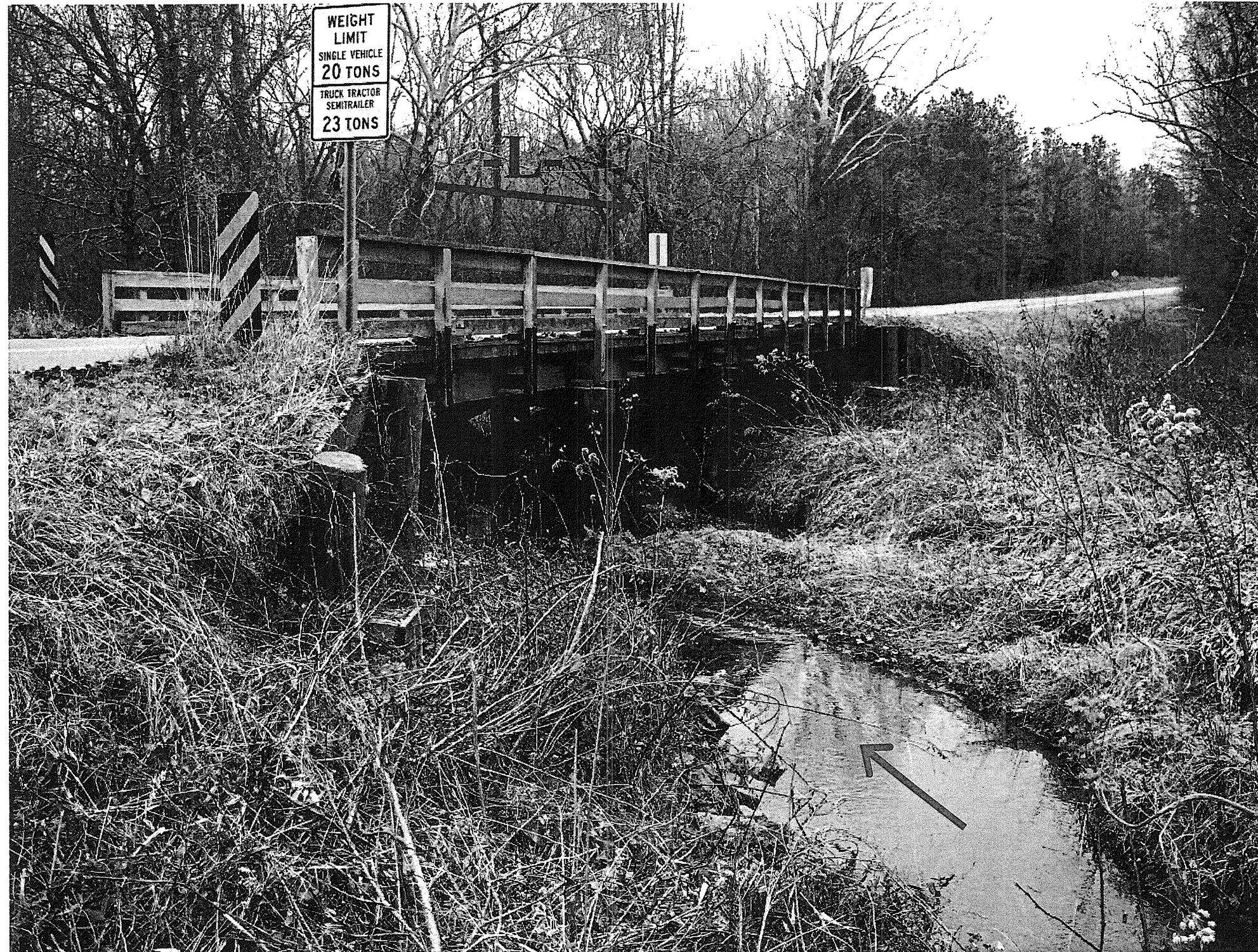
Looking North towards End Bent 2
