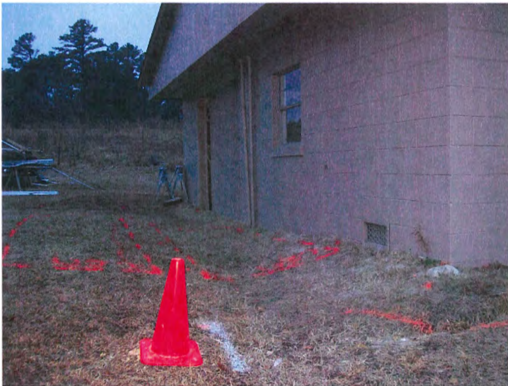
Photo #1: Location of probable USTs and Boring B-1 at south corner of building.
