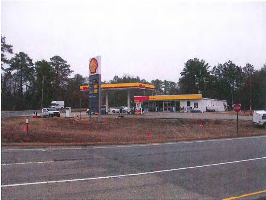
Photo #1: Overall view of the site looking east
