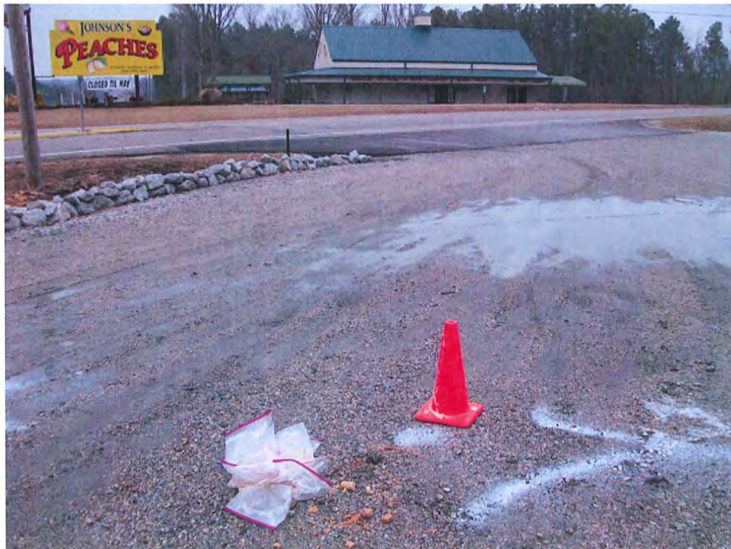
Photo #4: Location of Boring B-7 looking northwest
