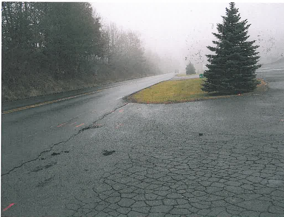
Photograph 2 View of the proposed right-of-way from northwest looking southeast.
