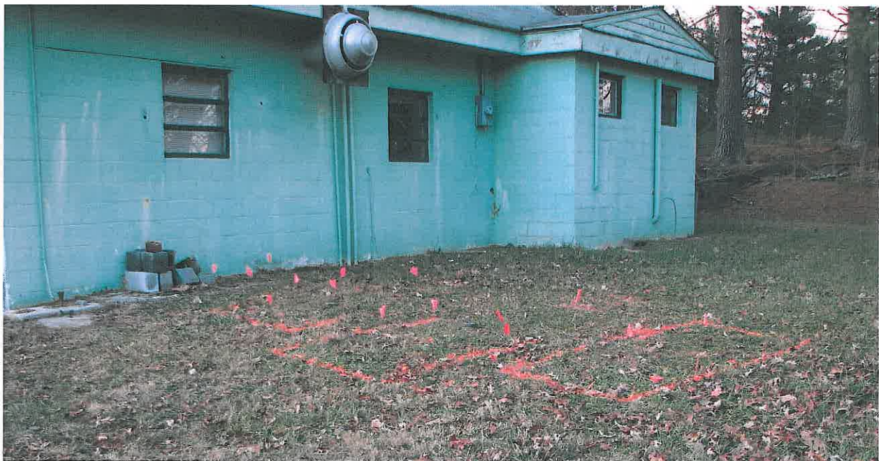
Photograph 2 – View of the three suspected USTs
