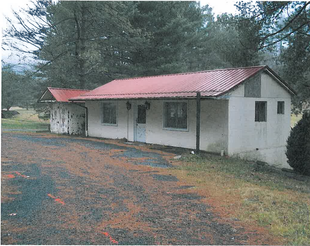
Photograph 1 View of the structures located onsite.
