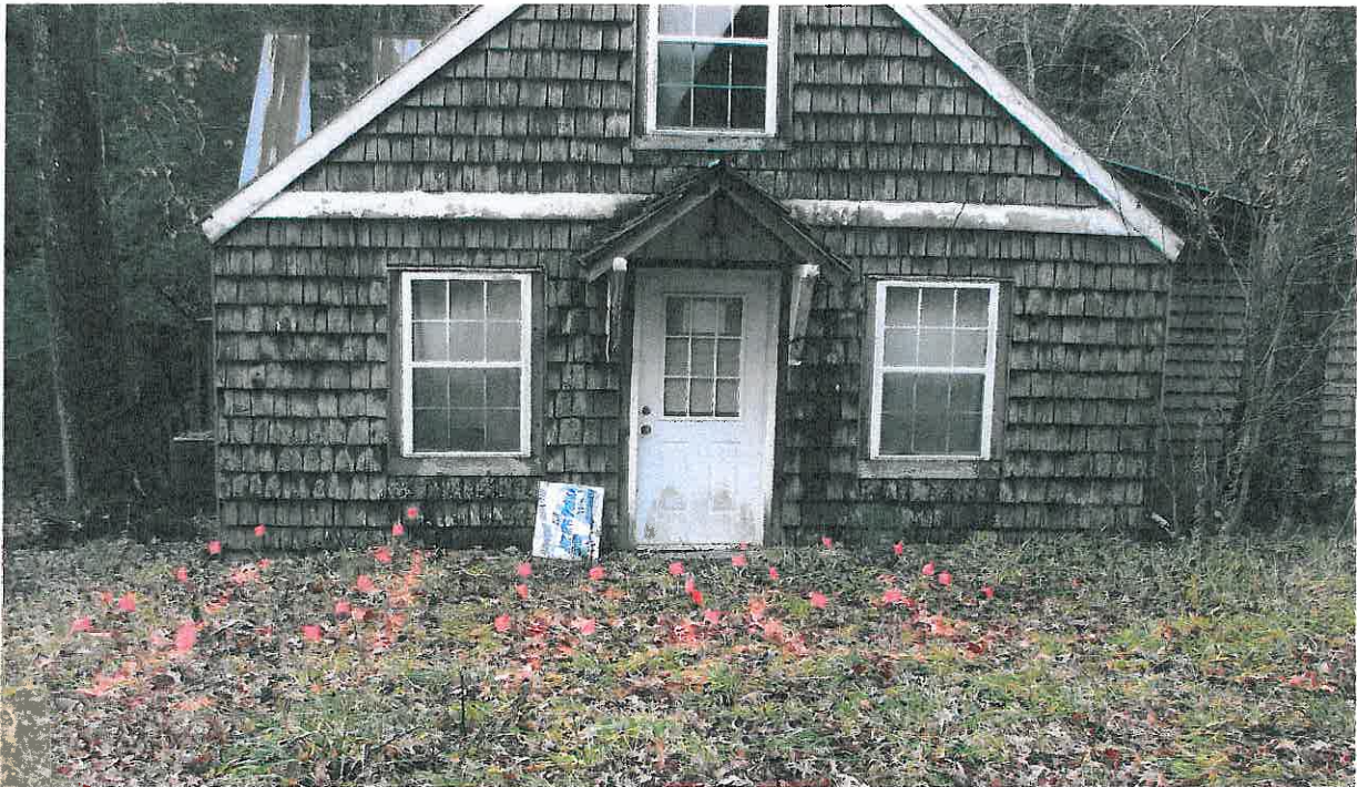
Photograph 1 – View of the former EJ Antiques building (currently vacant) looking south. The suspect UST field is located in the center of the photograph.
