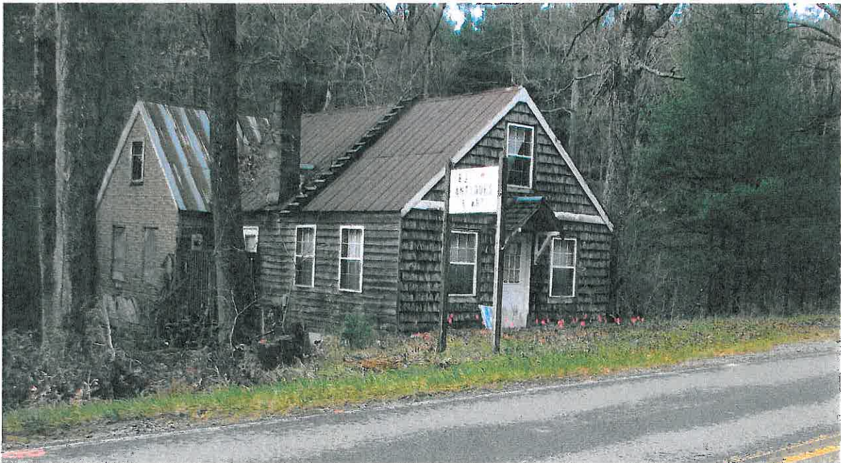
Photograph 2 – View of the building looking southwest.
