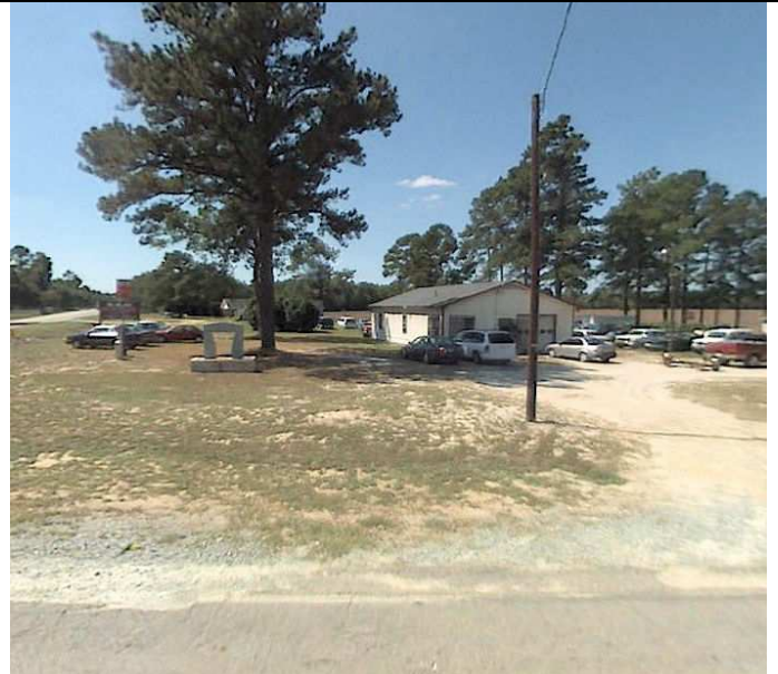
Site 4: Parcel 42. Miller Heating & Air Conditioning. View to the southwest.
