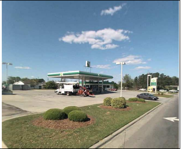
Site 14: Parcel 184. Han-Dee-Hugo's #8. View to the northeast.
