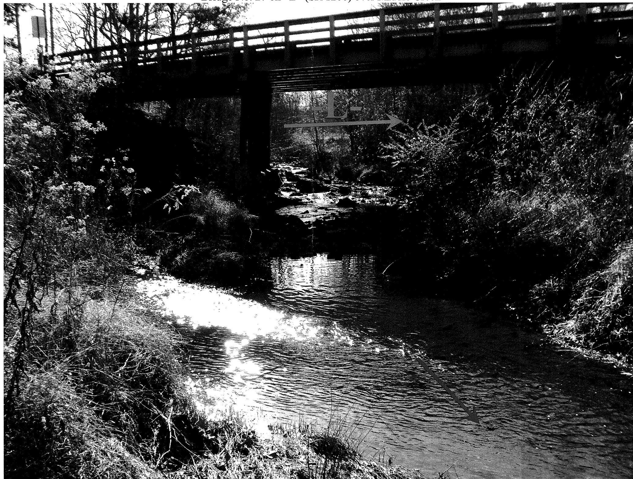
Bridge No. 27 on -L- (SR 1200) over Middle Creek
