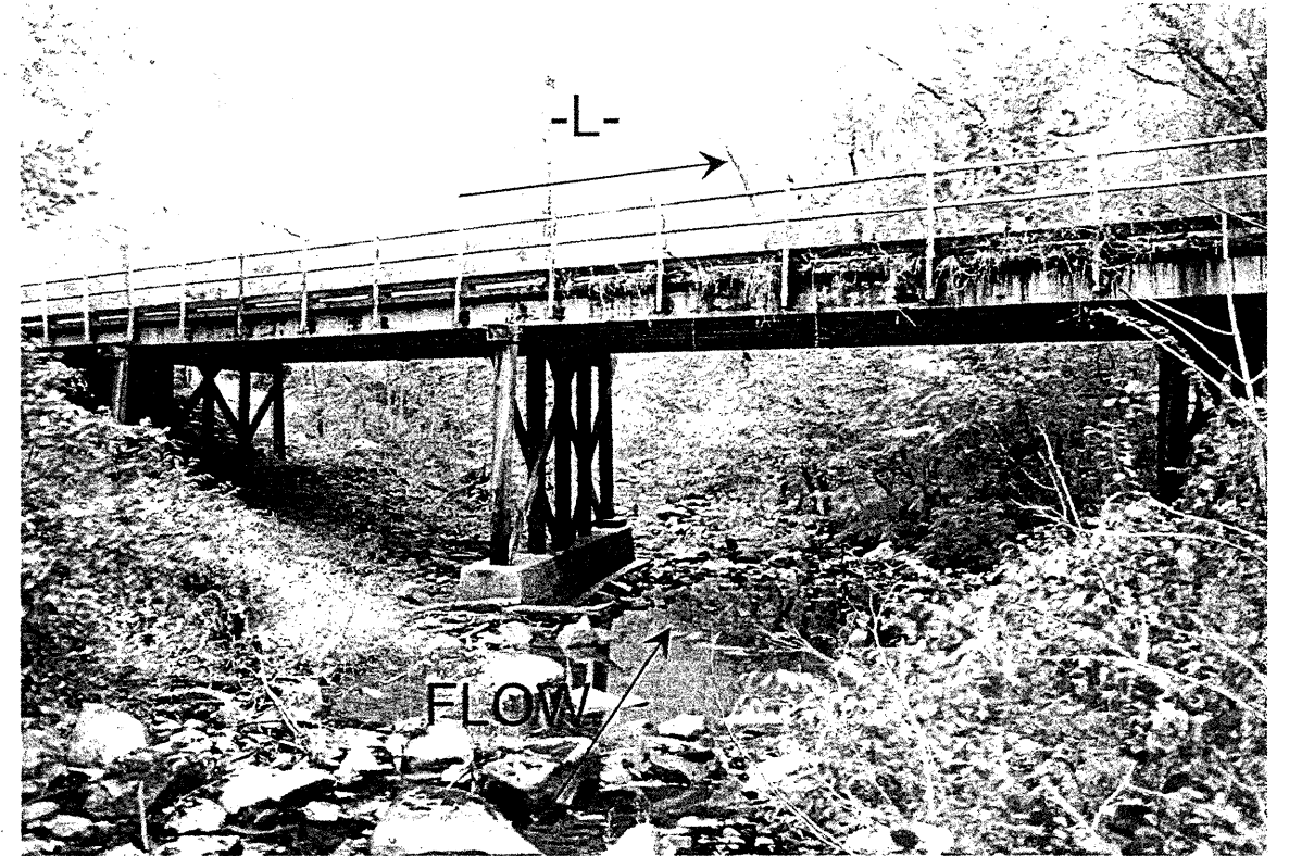
Existing Bridge No. 161, looking down stream
