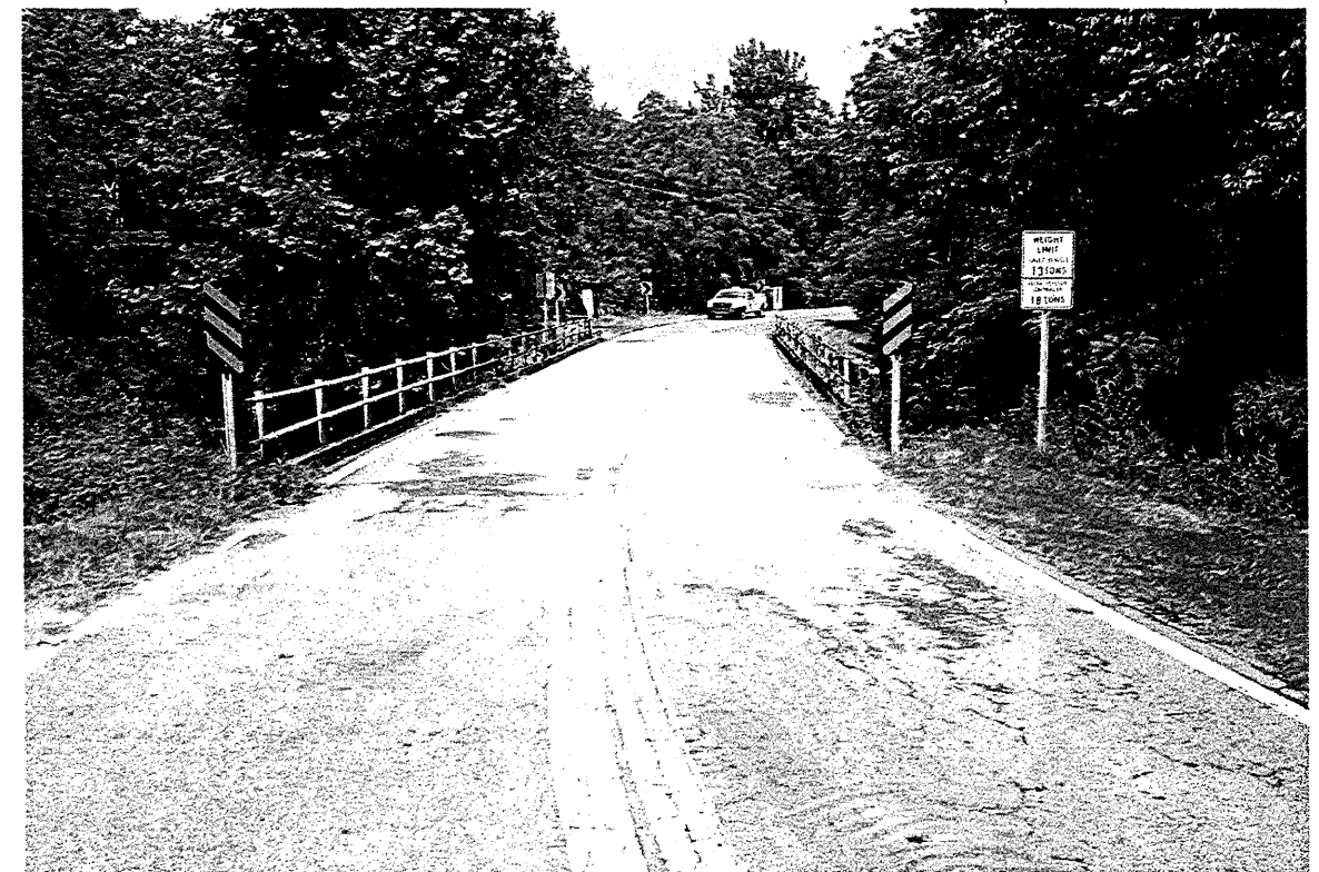
Center Line -L- looking down station
