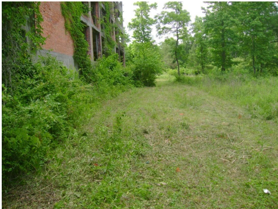
Parcel 59A – D&G Properties of Wilmington, LLC, looking southeast after clearing
