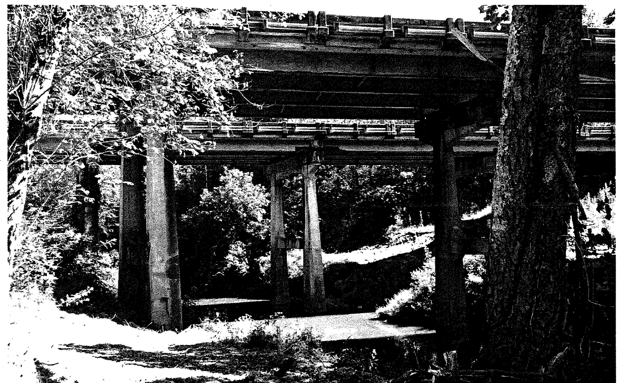
Interior Bents Looking Up-Stream
