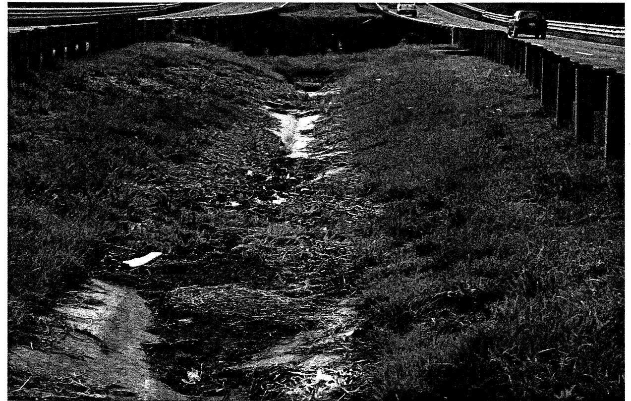
End Bent 1, Looking Southeast
