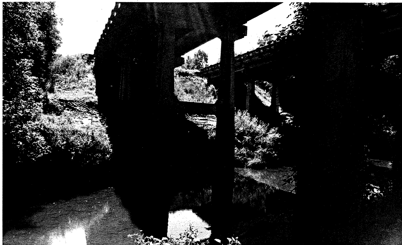
Interior Bents NBL Looking Southeast
