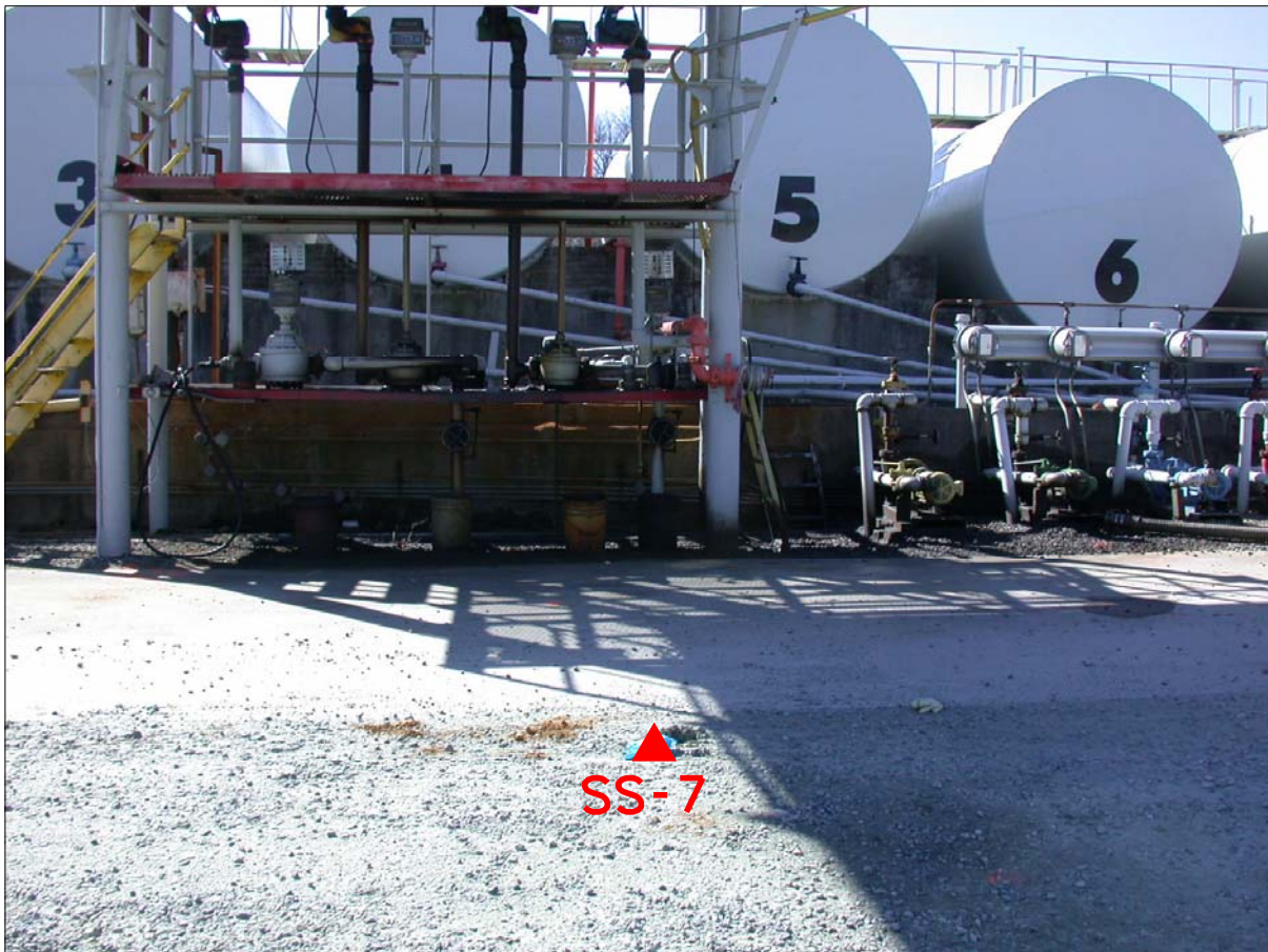
PHOTO 8 - BORING AT BULK FUEL LOADING PLATFORM LOOKING WEST
