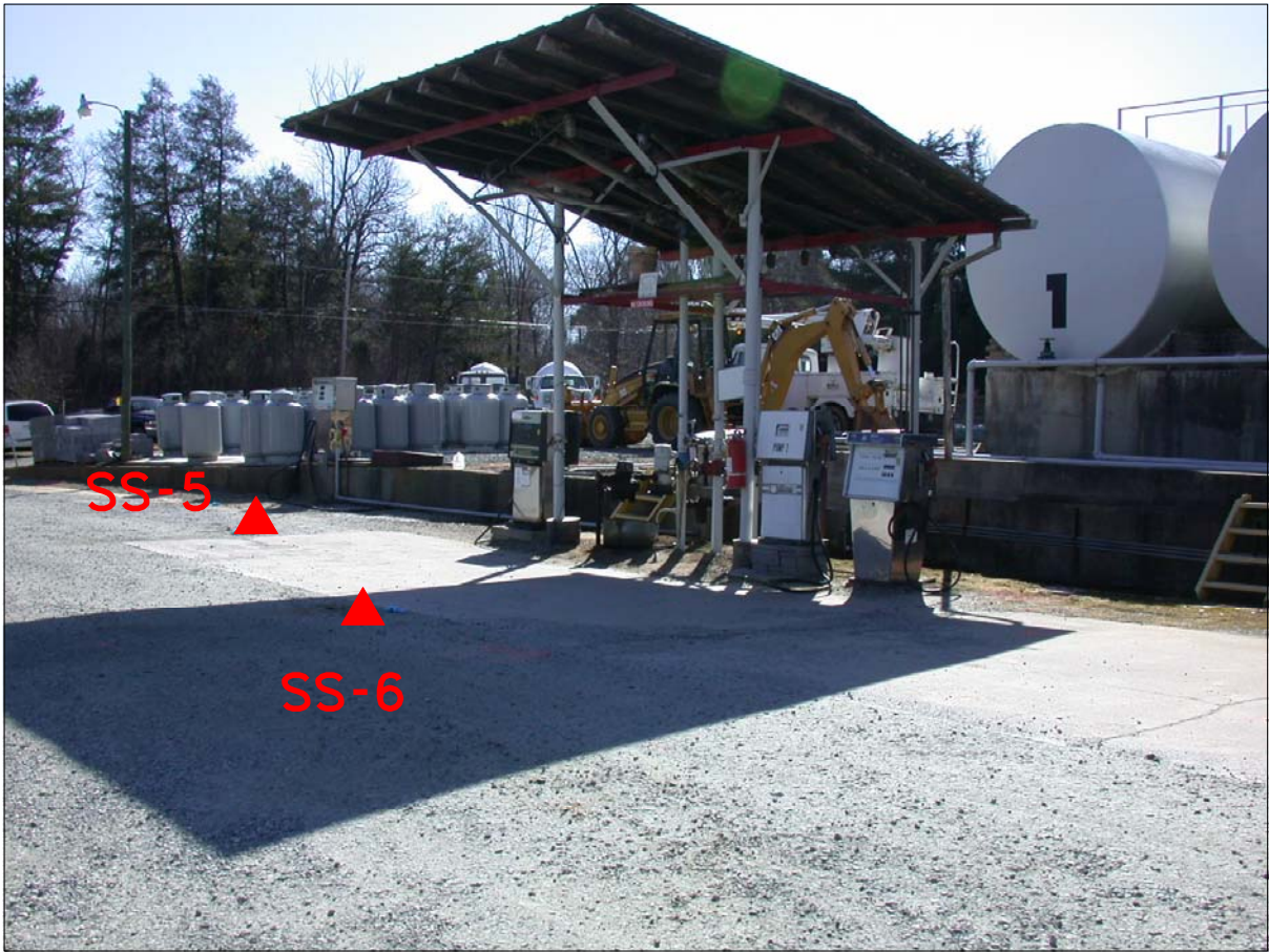
PHOTO 7 - BORINGS AT BULK FUEL DISPENSERS LOOKING SOUTH
