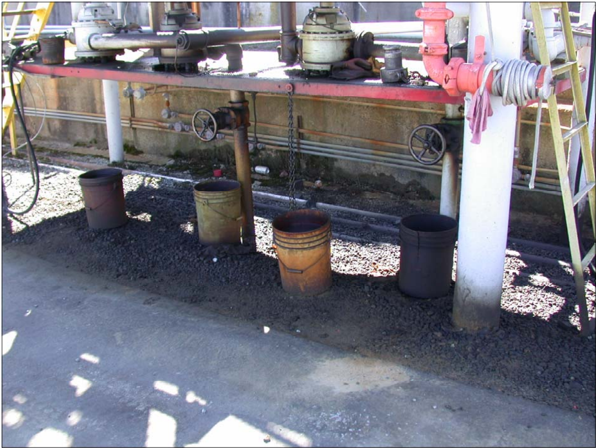
PHOTO 13 - SURFACE-STAINED SOIL AT BULK FUEL LOADING
