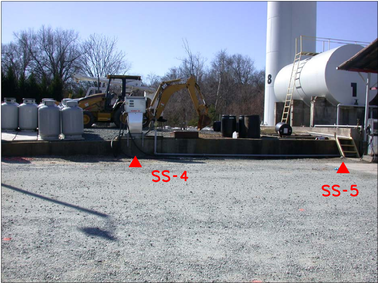
PHOTO 3 - BORING AT DIESEL FUEL DISPENSER LOOKING WEST
