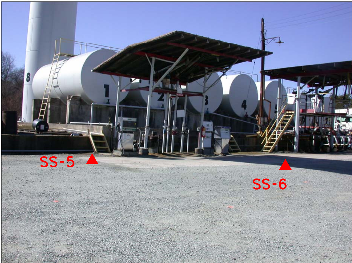
PHOTO 4 - BORINGS AT BULK FUEL DISPENSERS LOOKING NORTHWEST
