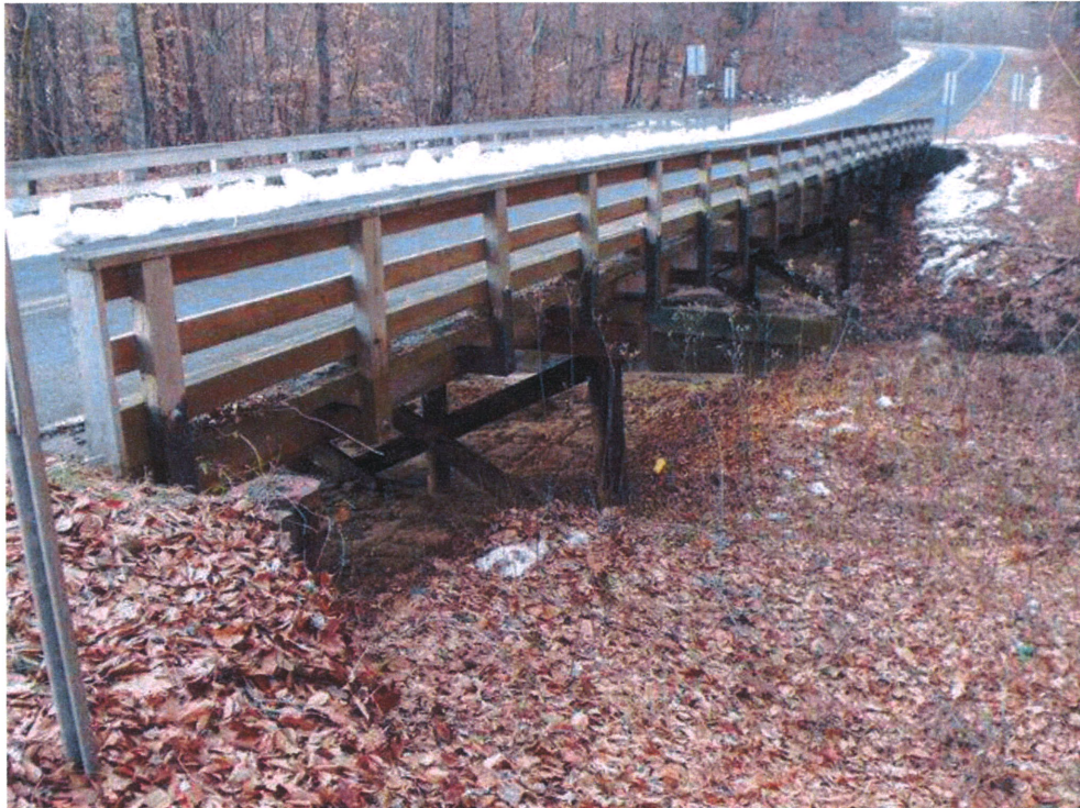
Looking east at existing structure
