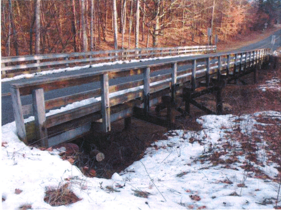
Looking west at existing structure
