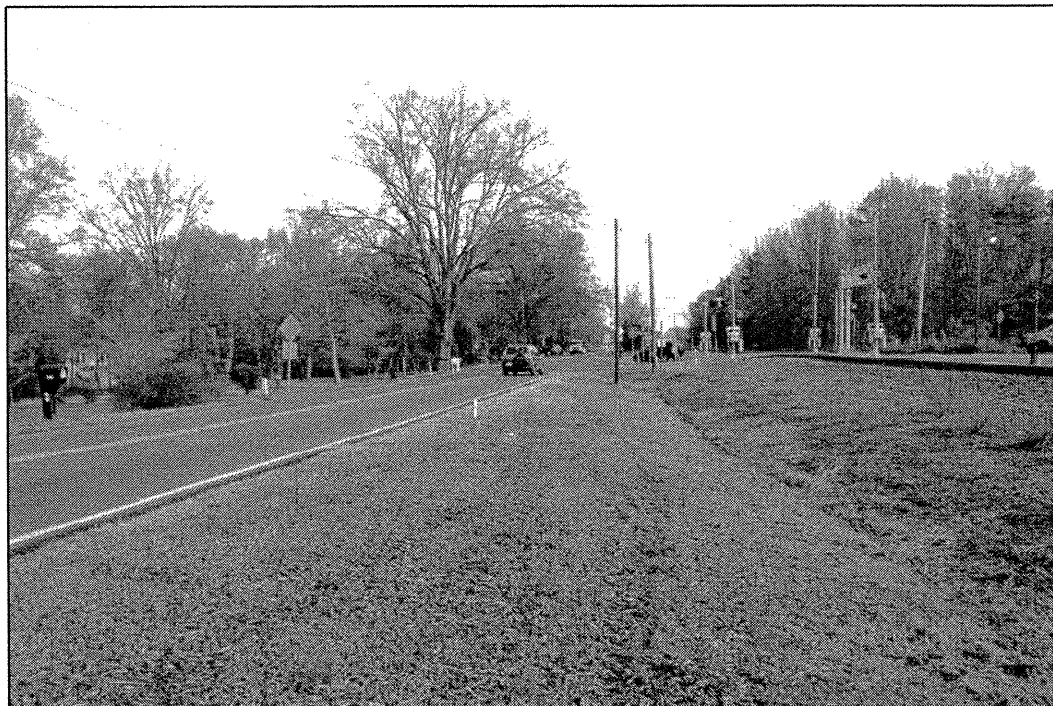
PHOTOGRAPH TAKEN FROM NEAR END OF RETAINING WALL LOOKING UPSTATION
