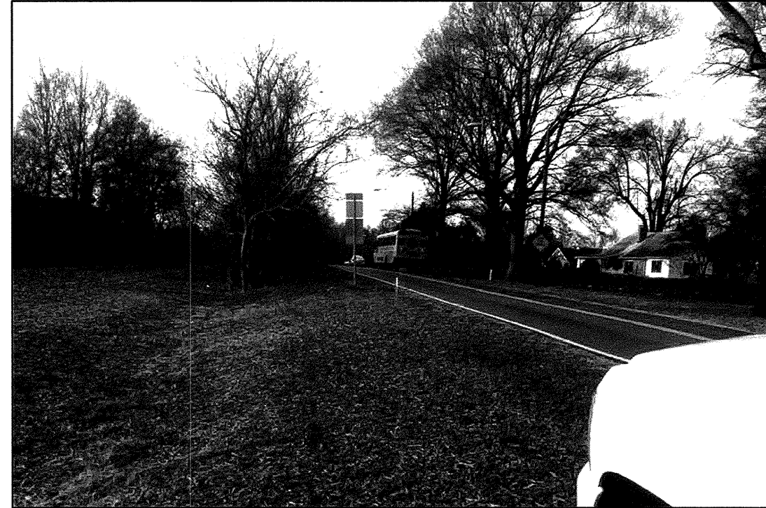
PHOTOGRAPH TAKEN FROM NEAR END OF RETAINING WALL LOOKING DOWNSTATION
