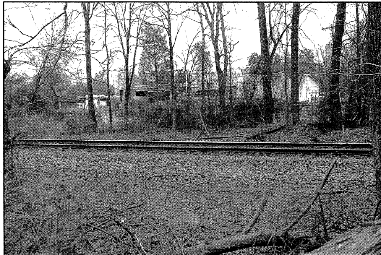
PHOTO TAKEN FROM NEAR END BENT 1, LOOKING UPSTATION (ALONG -L-) TOWARD B1-A (LEFT) AND B1-B (RIGHT), BEYOND EXISTING RAIL LINE SHOWN ABOVE.
