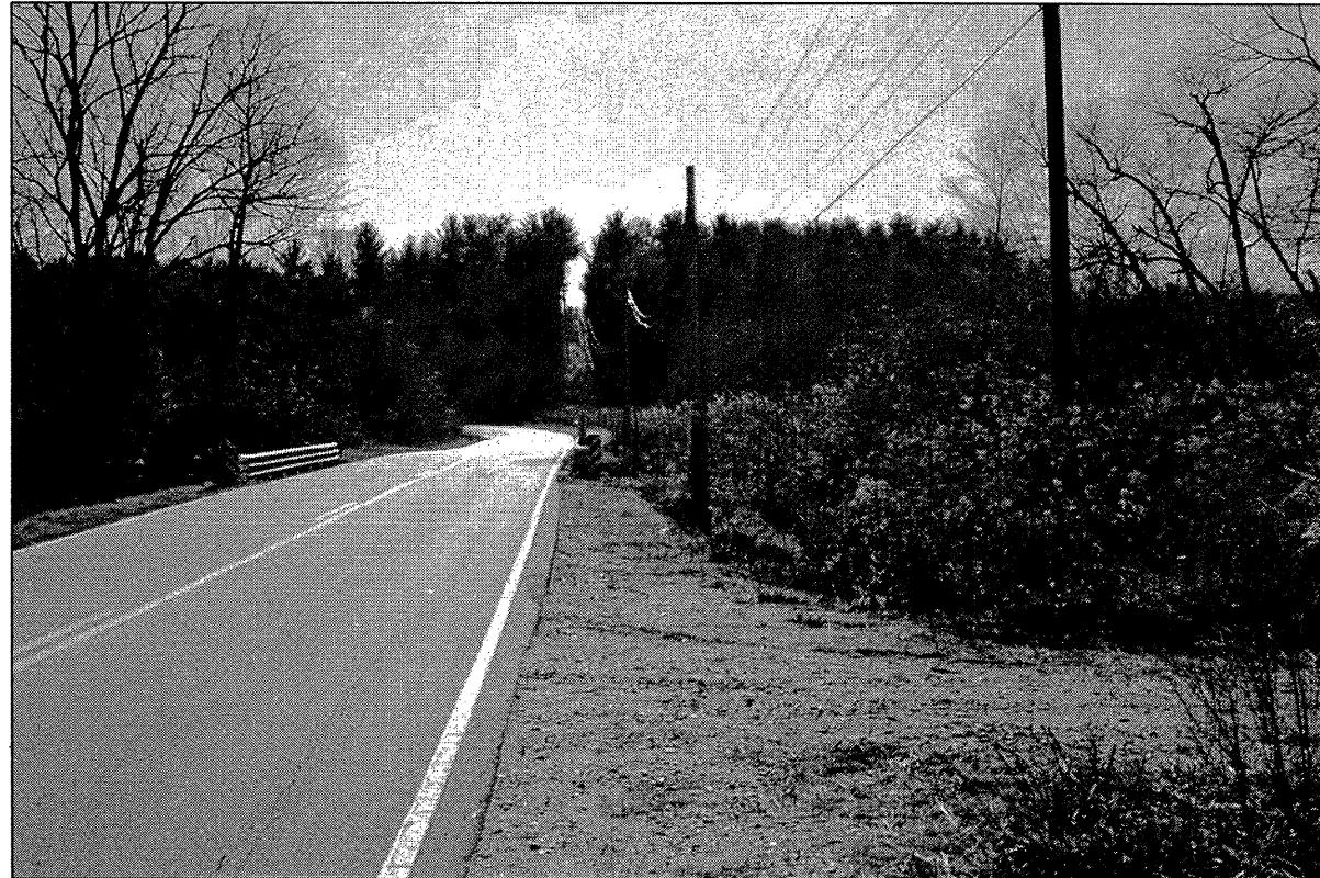
PHOTO TAKEN NEAR STATION 52+50 LOOKING DOWNSTATION.
