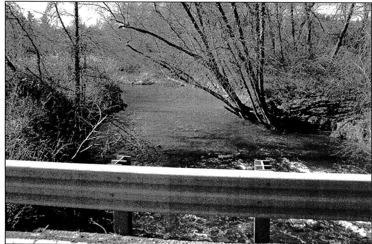
PHOTO TAKEN STANDING ON EXISTING BRIDGE LOOKING DOWNSTREAM.
