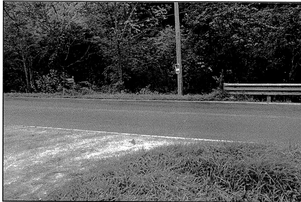
PHOTO 3: END BENT 1, LOOKING FROM RIGHT TO LEFT.
