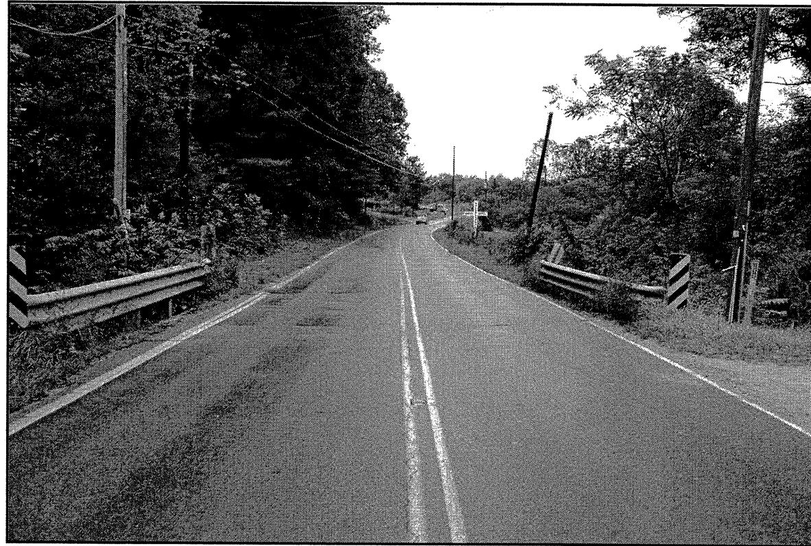
PHOTO 1: CENTERLINE PROFILE (-L-), LOOKING UPSTATION.
