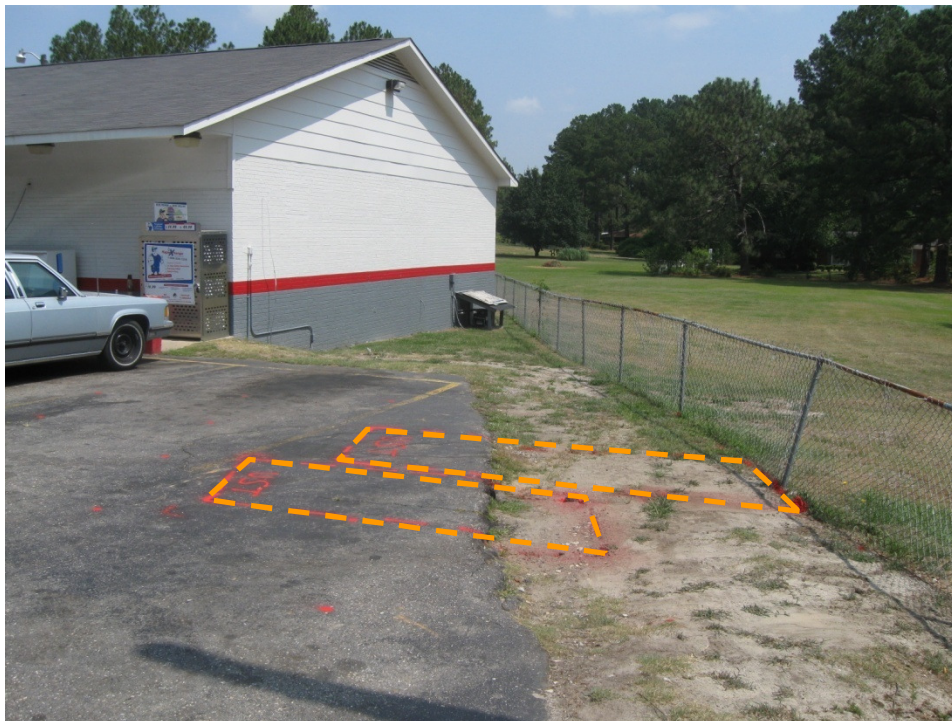
Parcel 4 – Leiburn R. Strickland Property, looking north. Photo shows approximate marked location of the two probable USTs on the southeast side of the property.
