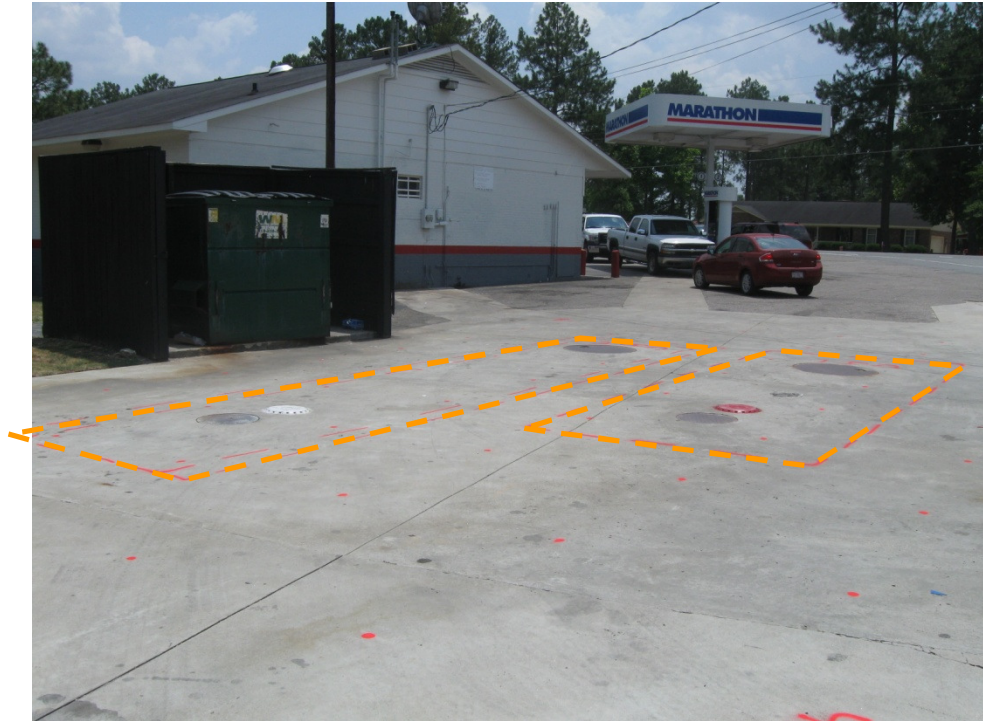
Parcel 4 – Leiburn R. Strickland Property, looking south. Photo shows approximate marked location of the two known USTs on the northwest side of the property.
