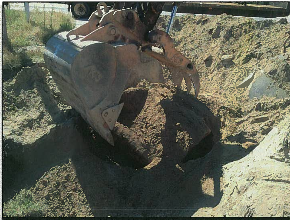
Looking South across Orphan UST basin.
