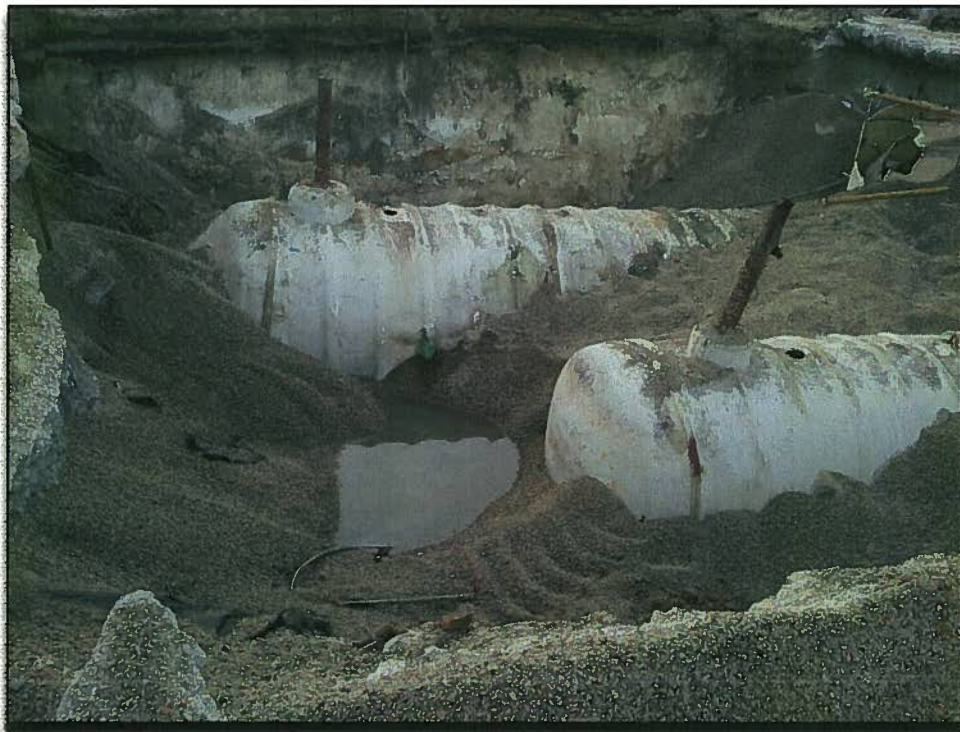
Looking East across UST #1 and UST #2 excavation.
