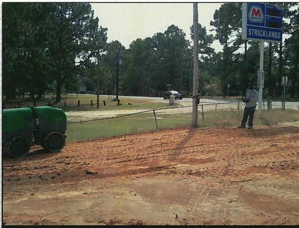
Orphan UST Basin backfilled and compacted.
