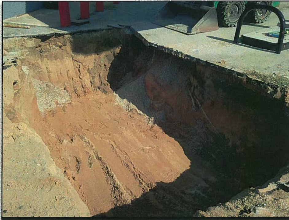
Looking East across proposed drainage feature excavation Northwest of former dispenser.
