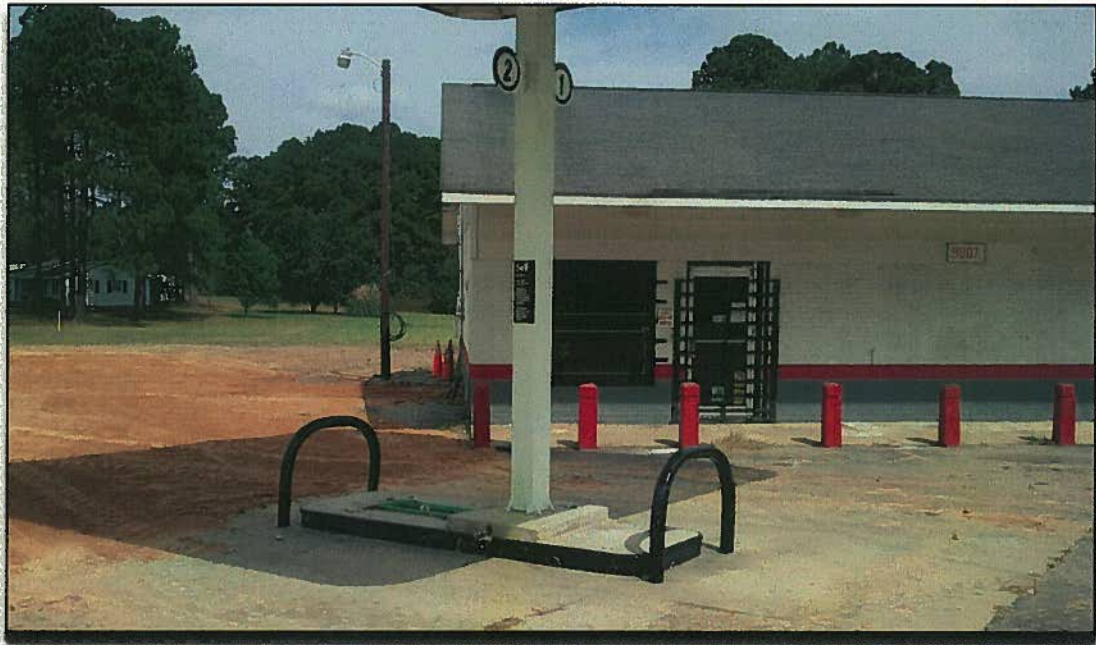
Looking North-northeast from near NC 24 after backfilling, compaction, and finish grading.
