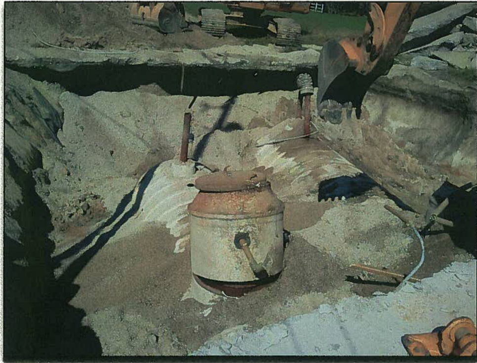
Looking North-northeast from south side of UST #1 and UST #2 excavation.
