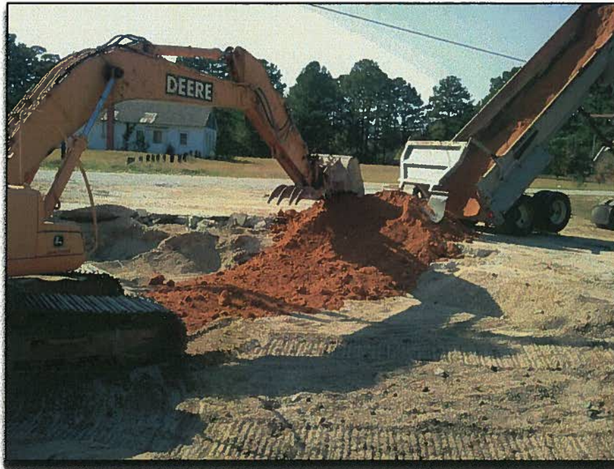
Looking East-northeast across UST basin being backfilled with off-site material.
