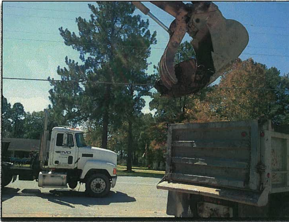
Orphan UST #1 being loaded for transportation off-site.
