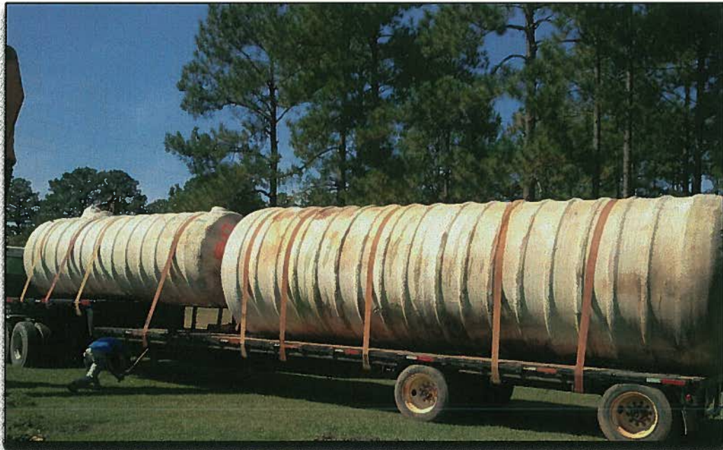
USTs #2 and #1 loaded (from left to right) for transportation off-site.
