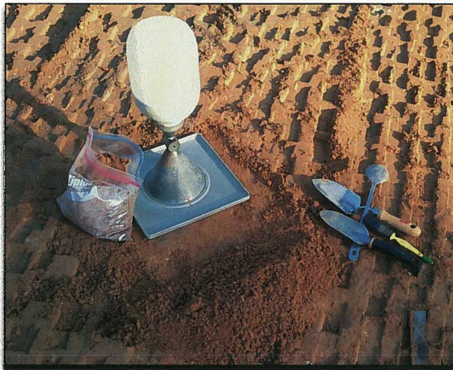
Excavation backfill sand cone compaction testing (typical).
