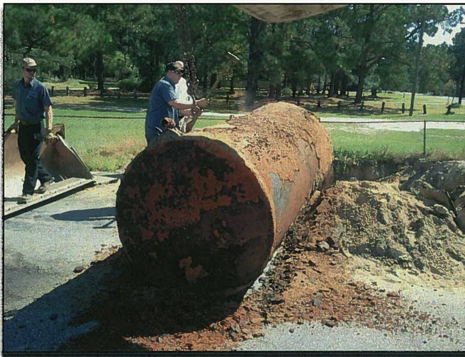
Looking East following Orphan UST #2 removal.
