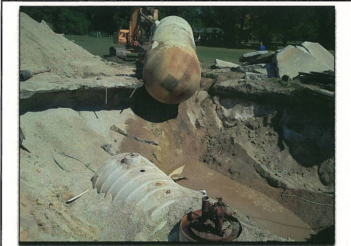
Looking Northeast across excavation, UST #1 being removed.
