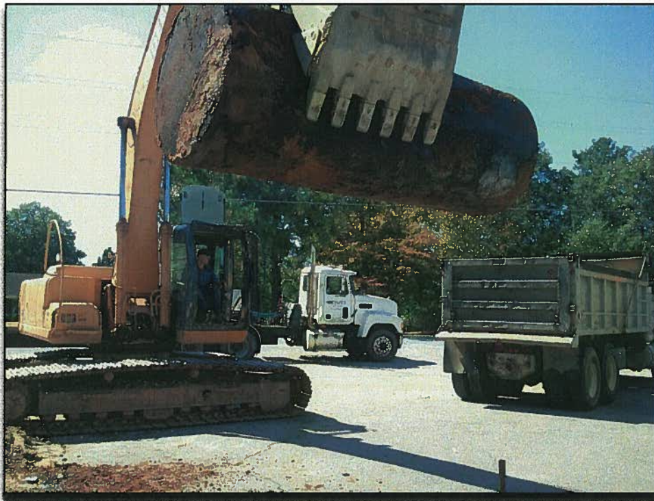
Orphan UST #2 being loaded for transportation off-site.
