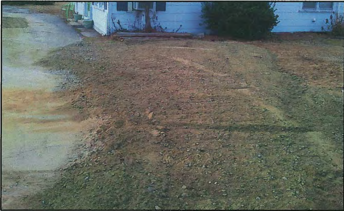
Looking West across backfilled UST #1 and UST #4 former locations.
