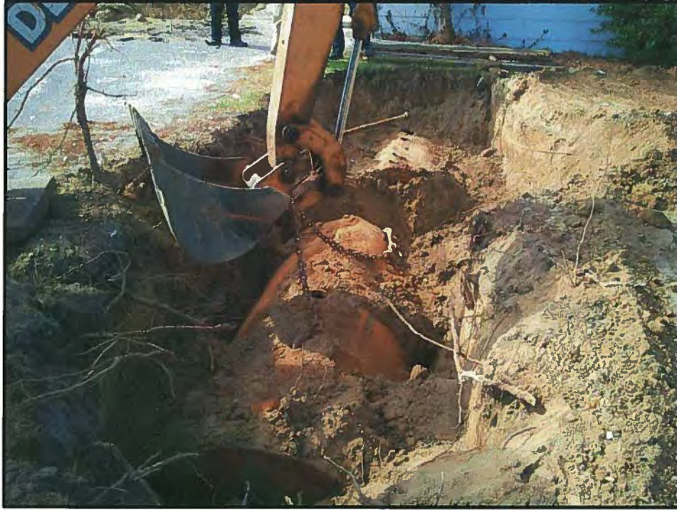
Looking West, UST #1 in background, UST #4 being removed.
