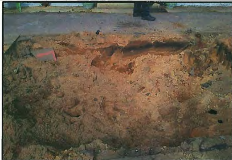
Looking North across former UST #2 (left) and former UST #3 (right) locations.
