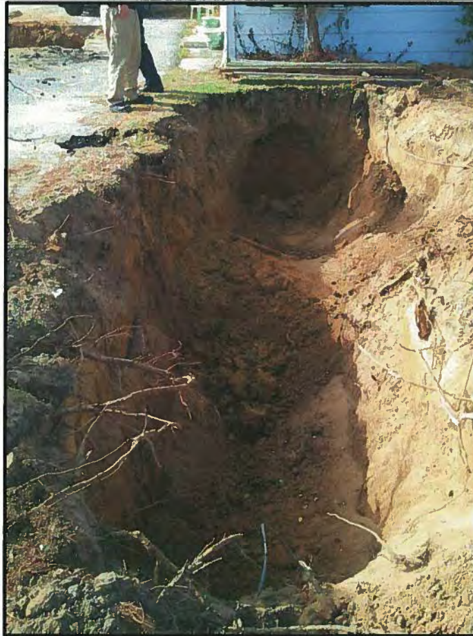
Looking West across former UST #4 (foreground) and former UST #1 (background) locations.
