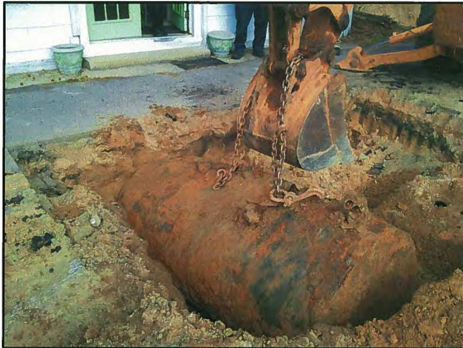
Looking Northeast, UST #3 on far right, UST #2 being removed.
