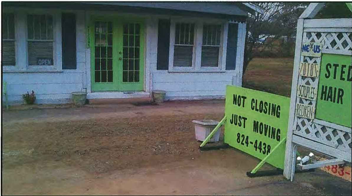
Looking Northeast across backfilled UST #2 and UST #3 former locations.
