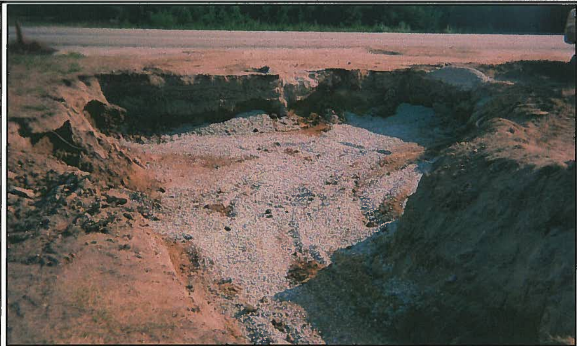
Looking South across UST #1, UST #2, and UST #3 excavation
