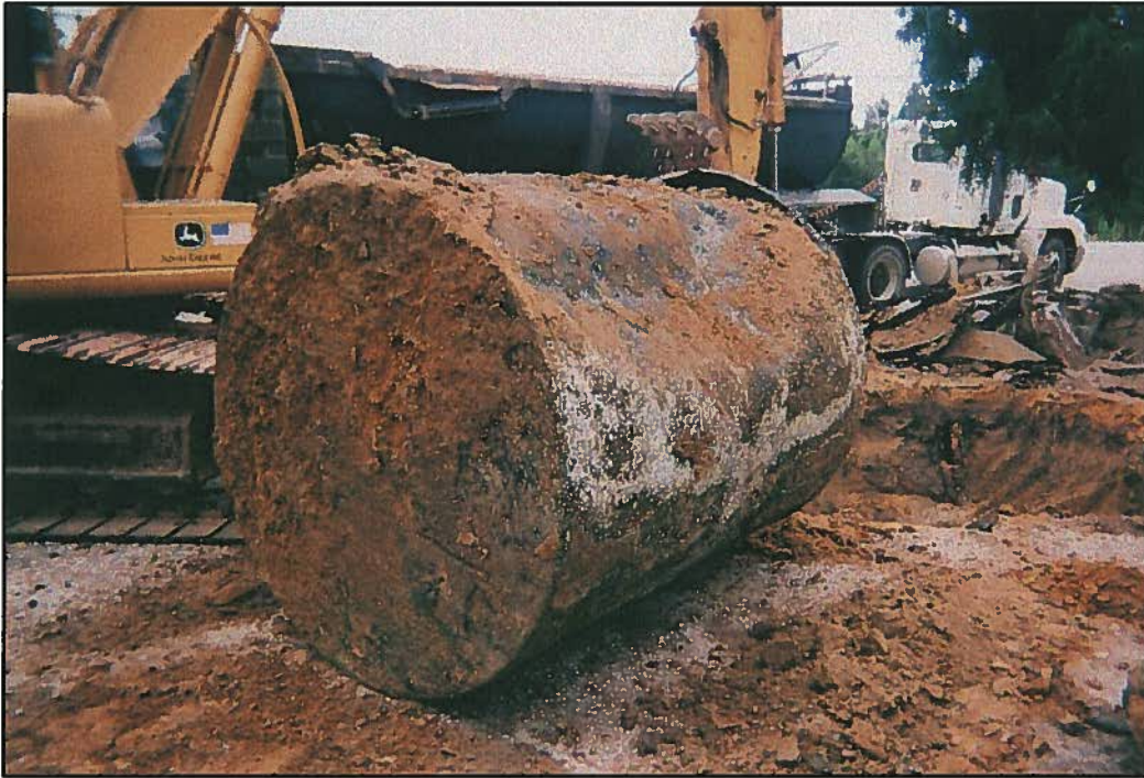
Looking South, UST #4 removed from excavation (in background).
