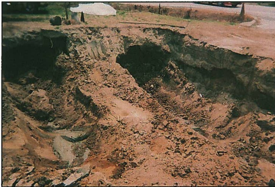
Looking East across UST #2 and UST #3 excavation.
