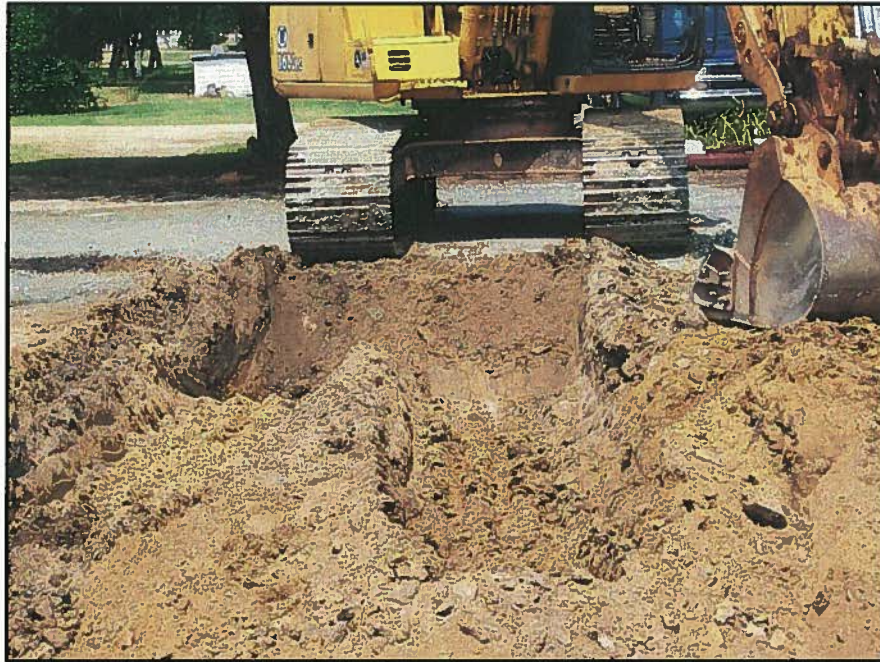
Looking East, Dispenser and line(s) excavation.
