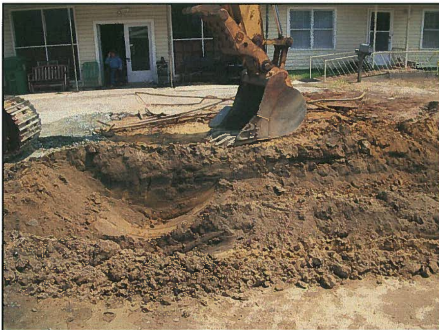
Looking North, Dispenser and line(s) excavation.
