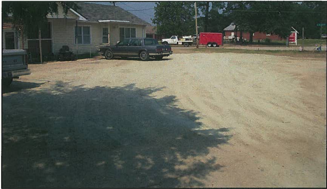
Looking Northeast across site after final backfilling and grading.
