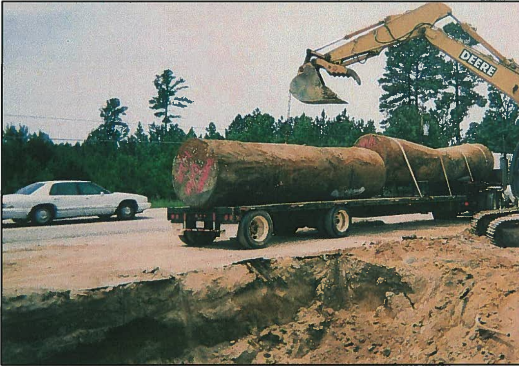
UST #2 and UST #3 loaded for transportation and disposal.
