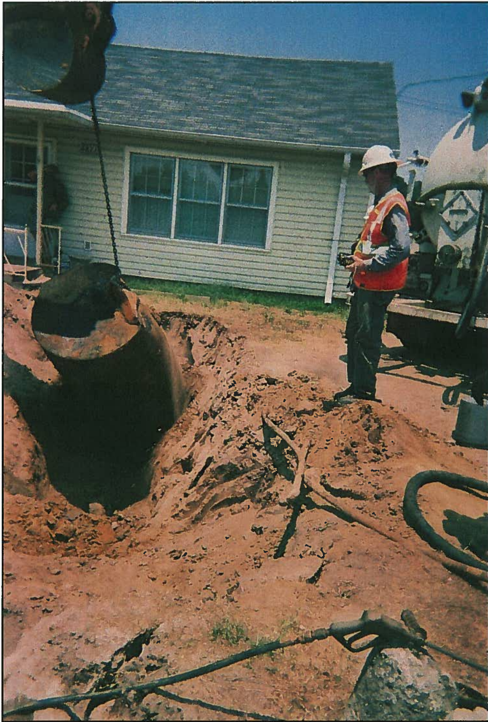
Looking North, UST #1 being removed.
