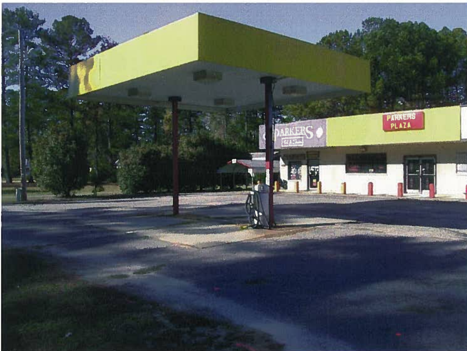
Parcel 71 – Harry T. Parker Property, looking northwest
