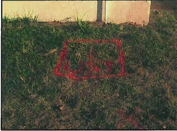
November 19, 2010 – Looking east, possible UST location identified during geophysical investigation near southwest corner of building.
