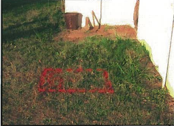
November 19, 2010 – Looking north, possible UST location identified during geophysical investigation near southwest corner of building.
