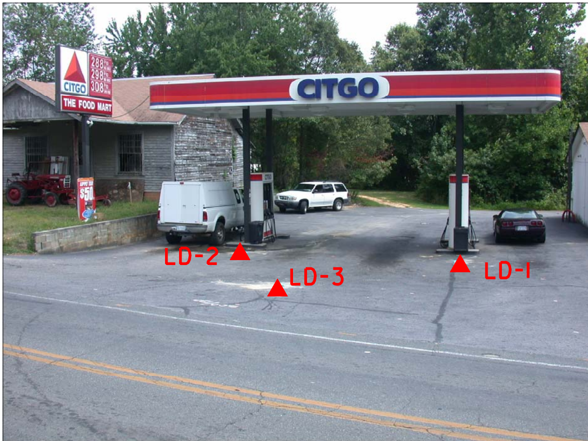
PHOTO 3 - BORINGS AT LUNSFORD PROPERTY LOOKING SOUTH FROM STREET
