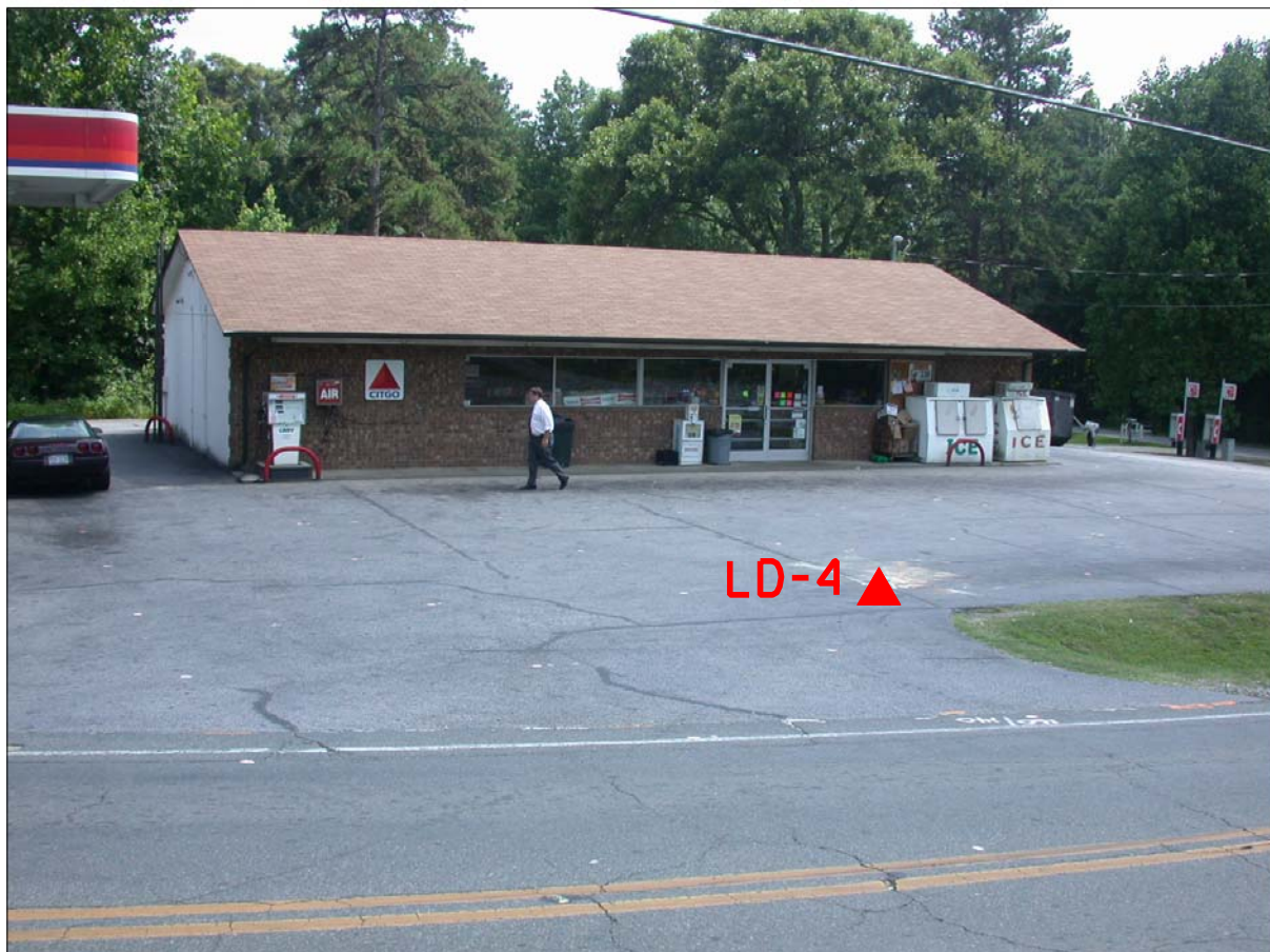
PHOTO 4 - BORINGS AT LUNSFORD PROPERTY LOOKING SOUTH FROM STREET
