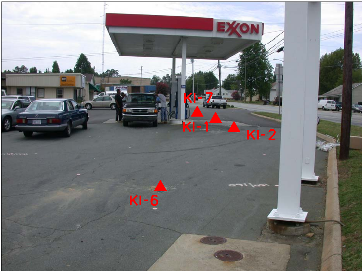
PHOTO 4 - BORING AT KING PROPERTY LOOKING SOUTH FROM SIGN
