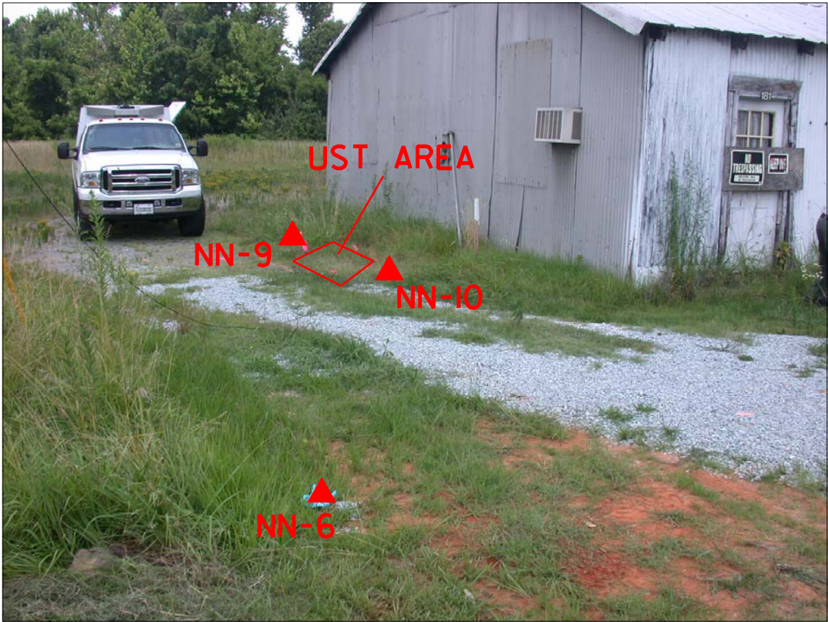
PHOTO 1- BORINGS AT HENDERSON PROPERTY LOOKING NORTH FROM STREET
