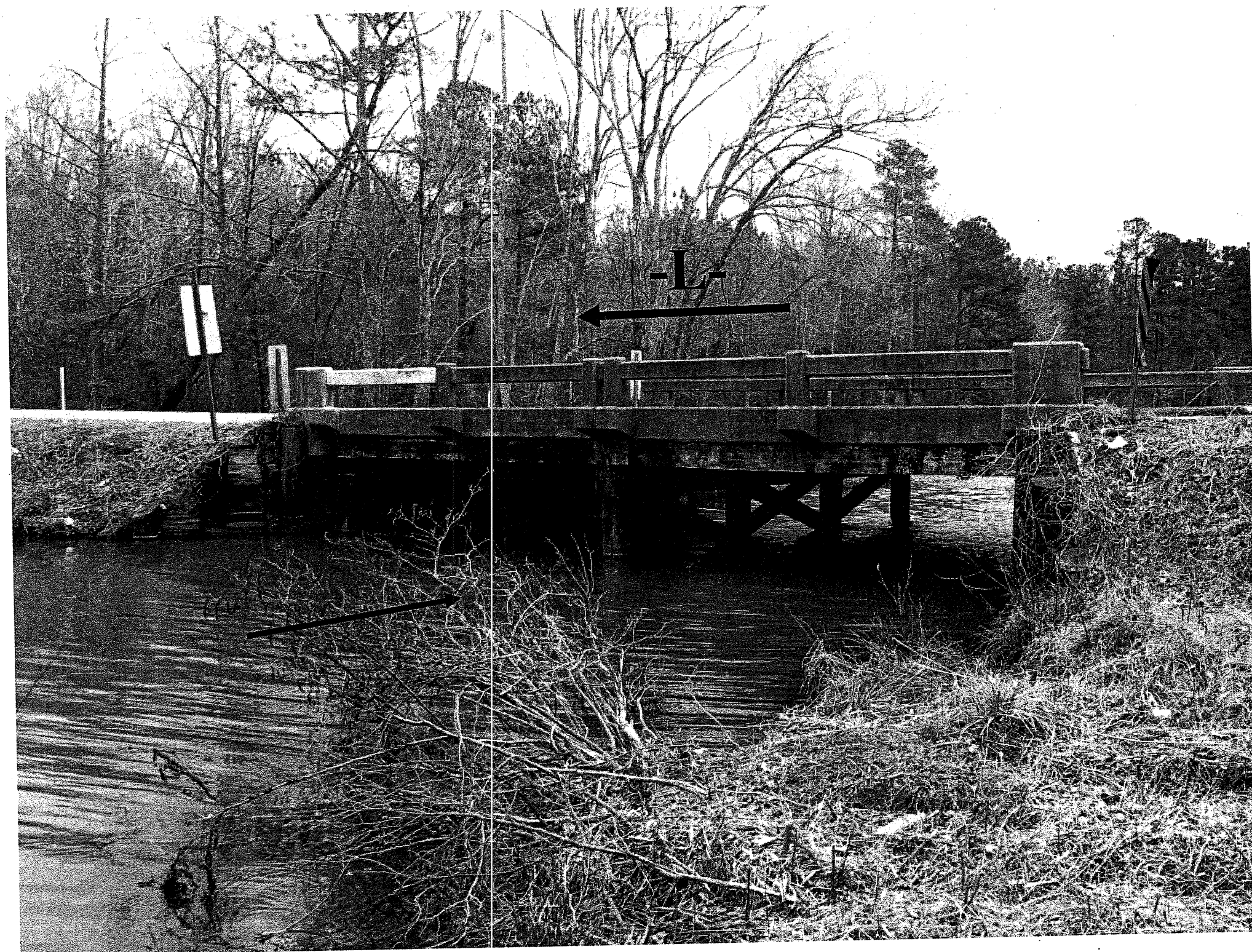
Looking South towards End Bent 2
