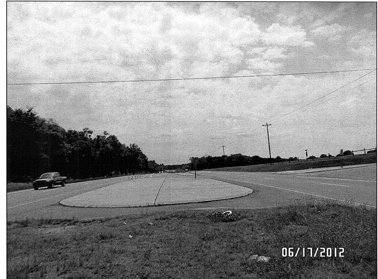
NC 49 (-Y4-) CROSSING AT STA. 25+40 -L-, LOOKING WEST
