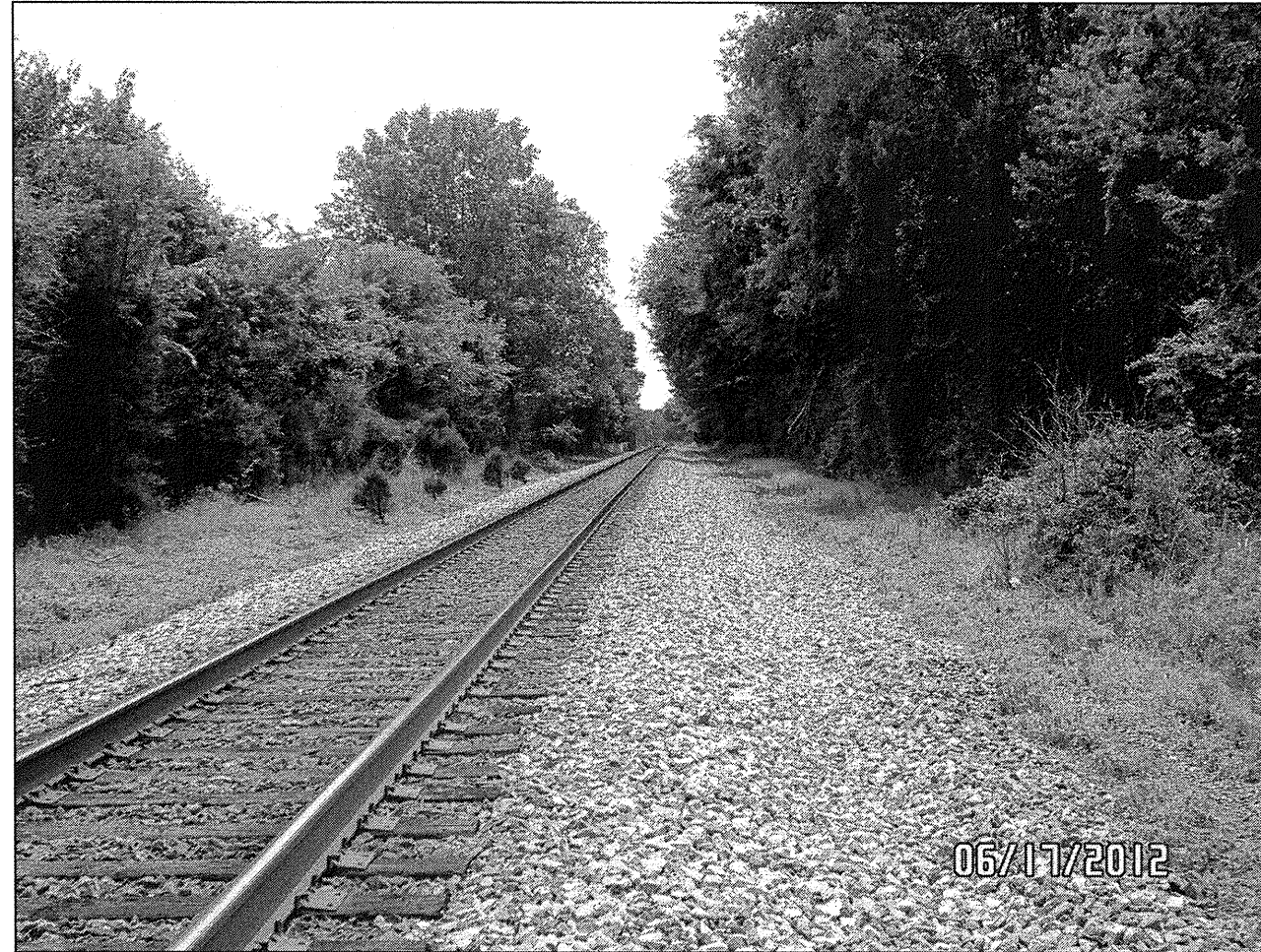
NCRR/NS CROSSING AT STA. 23+80 -L-, LOOKING WEST
