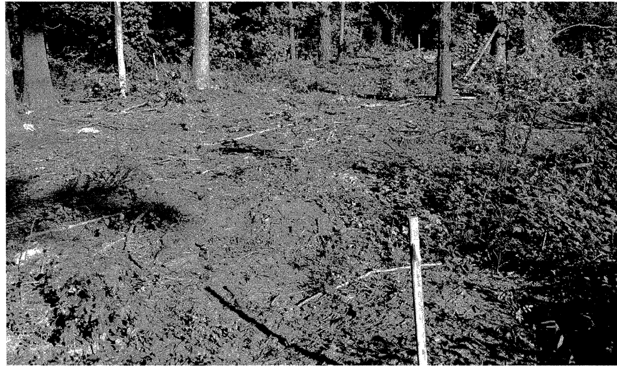
End Bent 1 Looking Northwest Toward Railroad & Main Street
