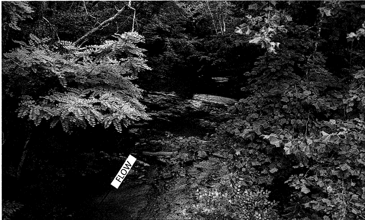
PHOTO TAKEN FROM EXISTING BRIDGE DECK FACING UP STREAM
