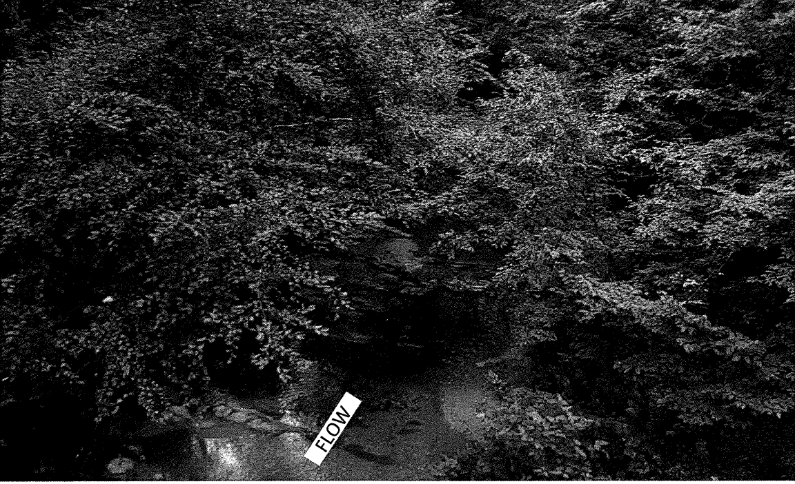
PHOTO TAKEN FROM EXISTING BRIDGE DECK FACING DOWN STREAM
