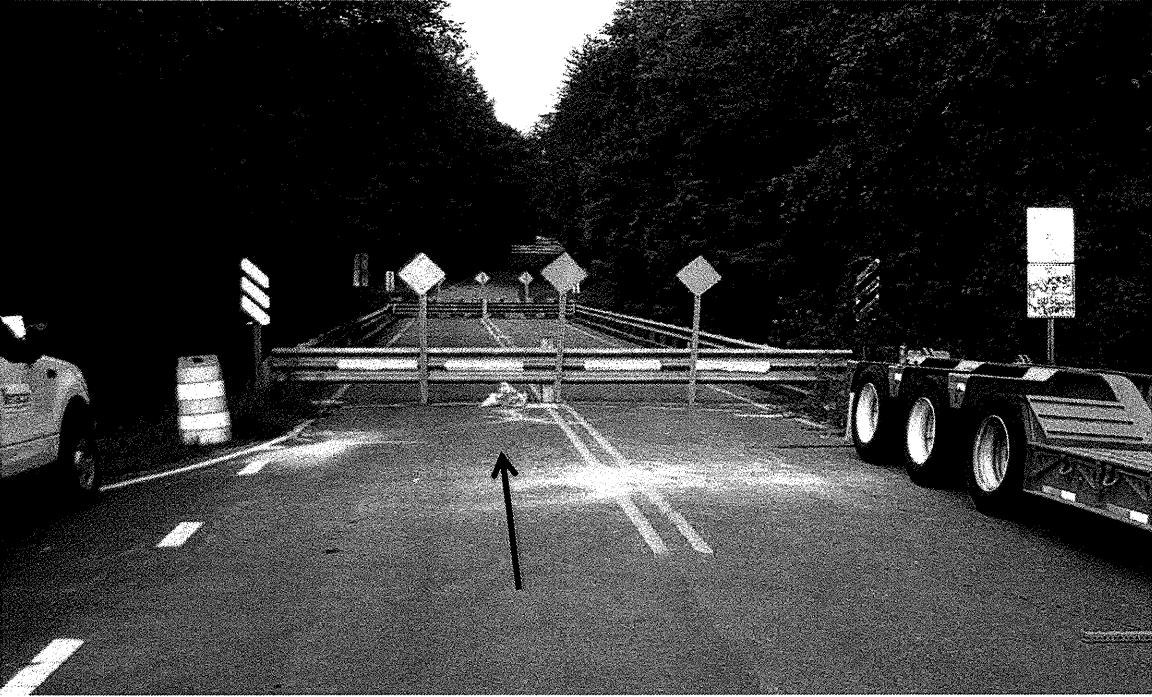
PHOTO TAKEN FROM DOWN STATION OF BRIDGE FACING UP STATION
