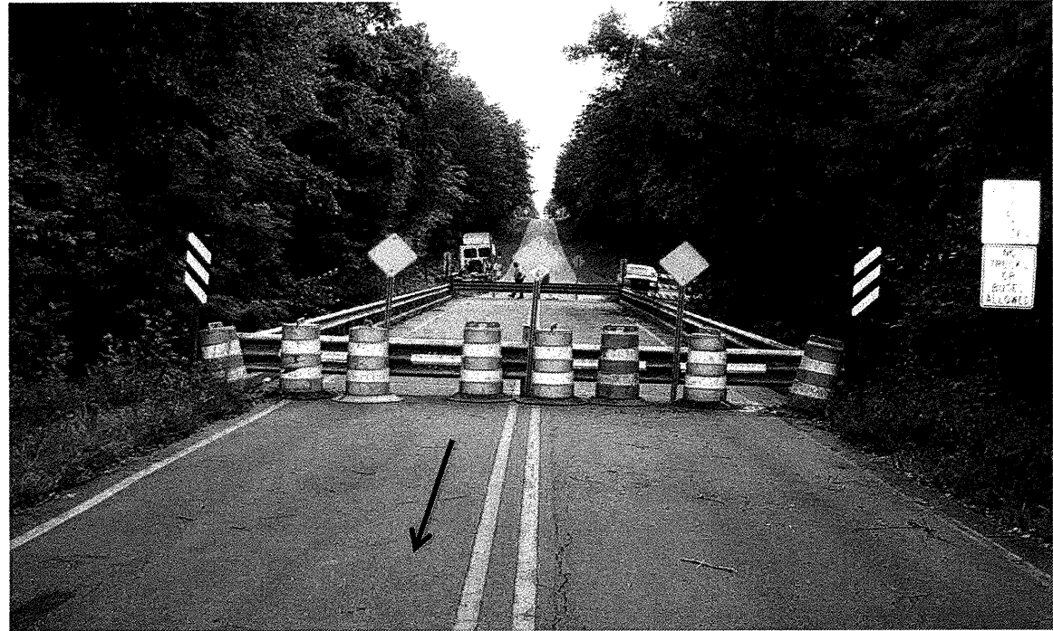
PHOTO TAKEN FROM UP STATION OF BRIDGE FACING DOWN STATION
