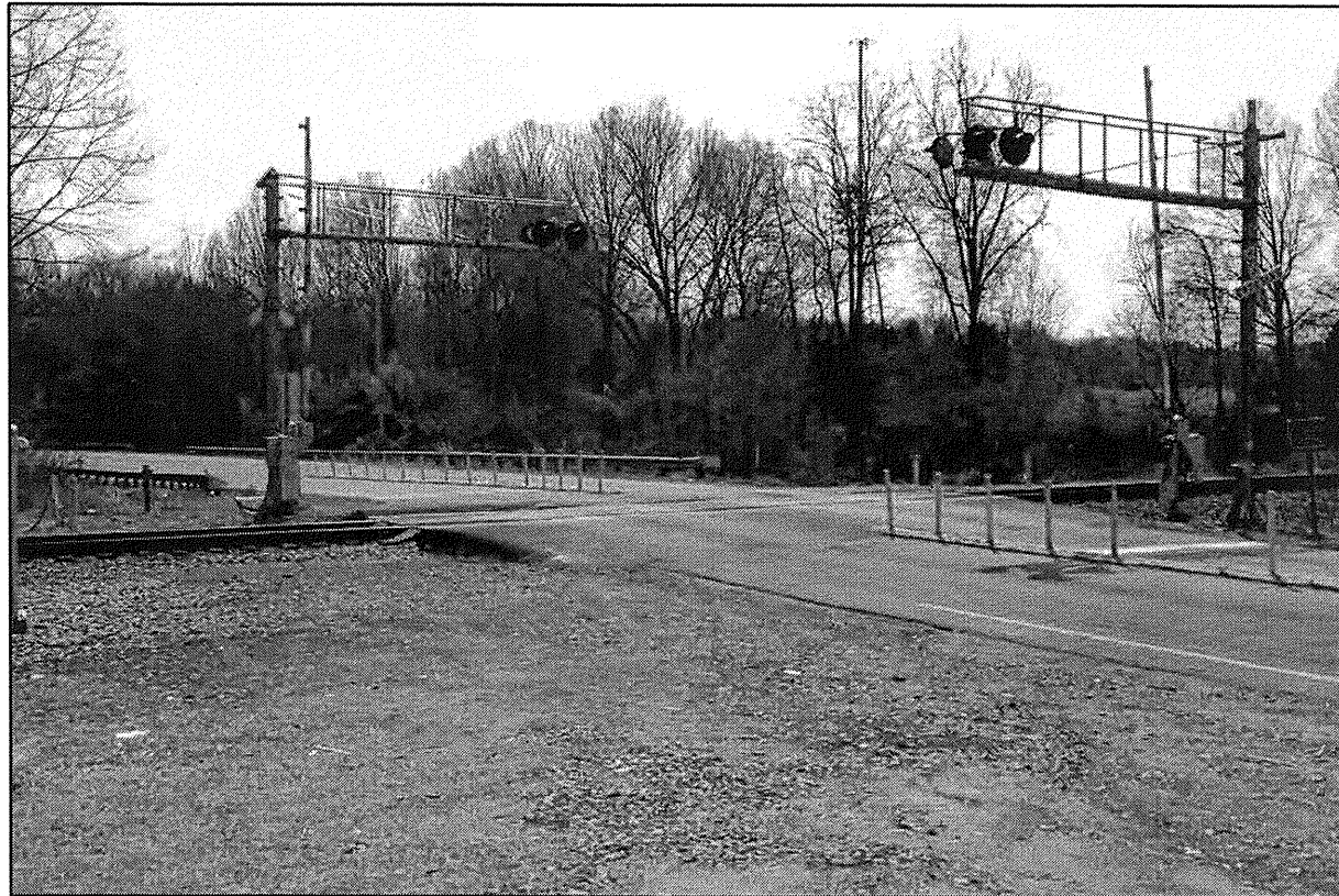
PHOTO 1: EXISTING AT-GRADE CROSSING, LOOKING SOUTHWEST FROM BETWEEN END BENT 1 AND BENT 1
