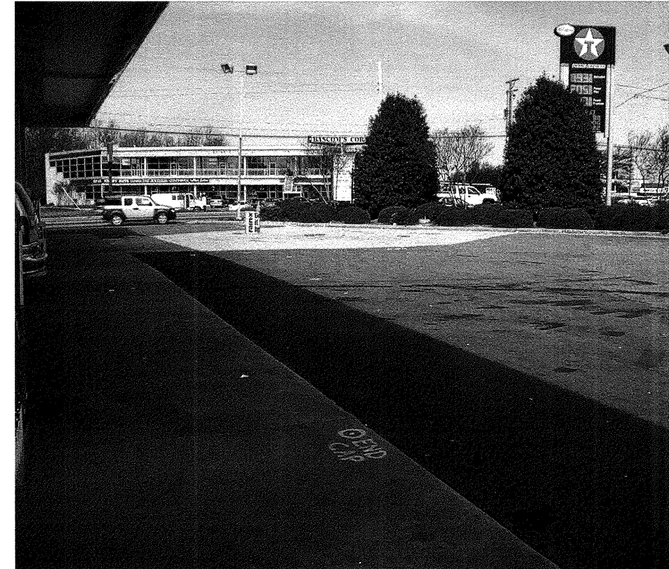
Photograph 3 – View Left to Right Across End Bent-2
