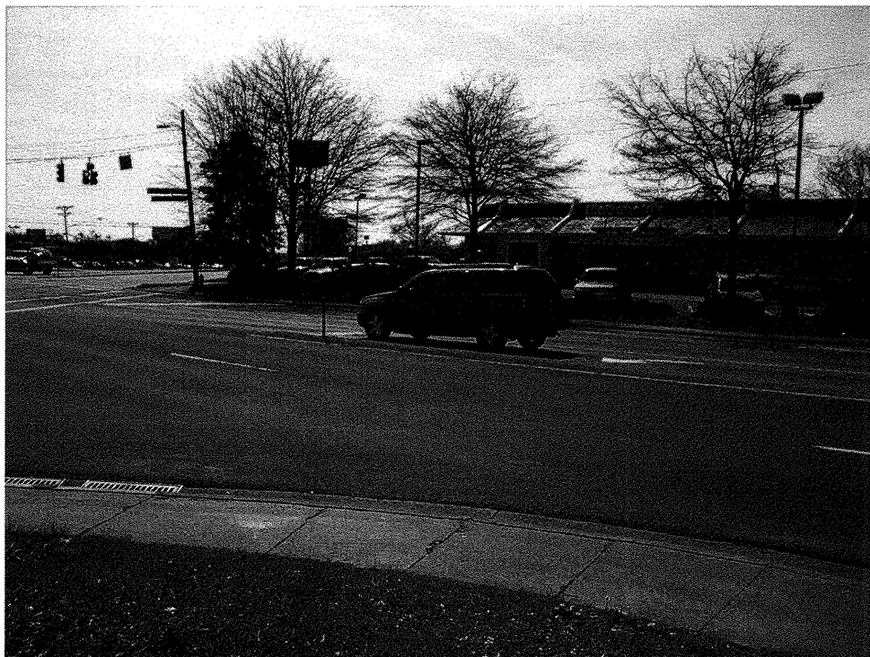
Photograph 2 – View Left to Right Across End Bent-1
