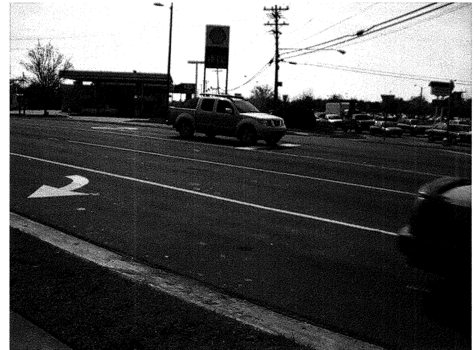
Photograph 4 – View Left to Right Across End Bent-2
