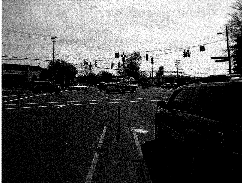
Photograph 1 – View Looking Upstation From EB1-C to EB2-C
