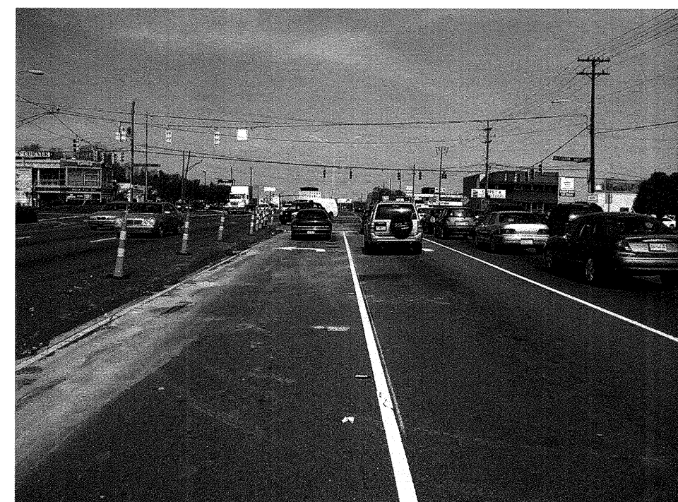
Photograph 4 – View Left to Right Across Bent-2
