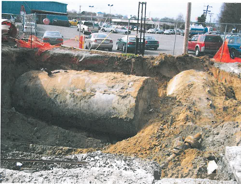
Photograph 8 – View of UST #1 and #2.
