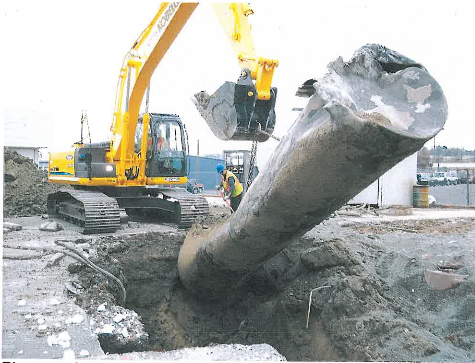
Photograph 5 – View of the removal of UST #5.
