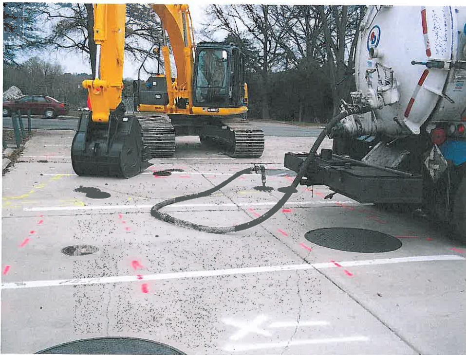
Photograph 4 – View of A&D vacuuming product from the USTs.
