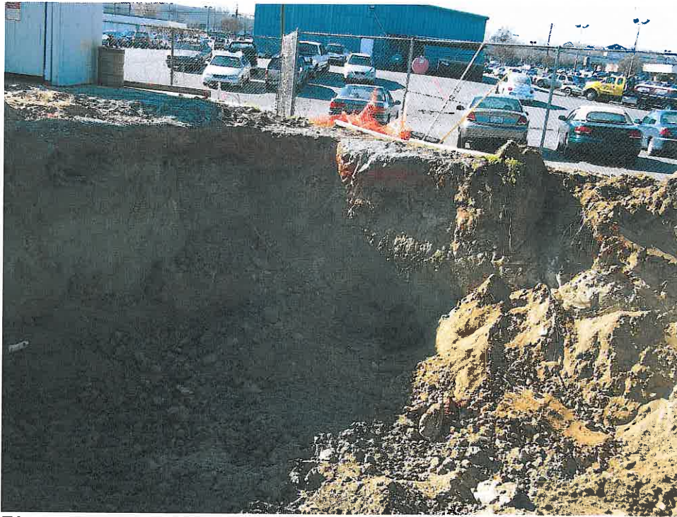
Photograph 11 – View of UST basin following the UST removal.
