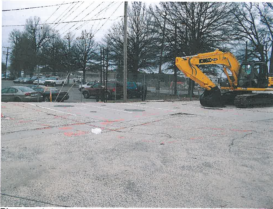
Photograph 3 – View of the UST basin.
