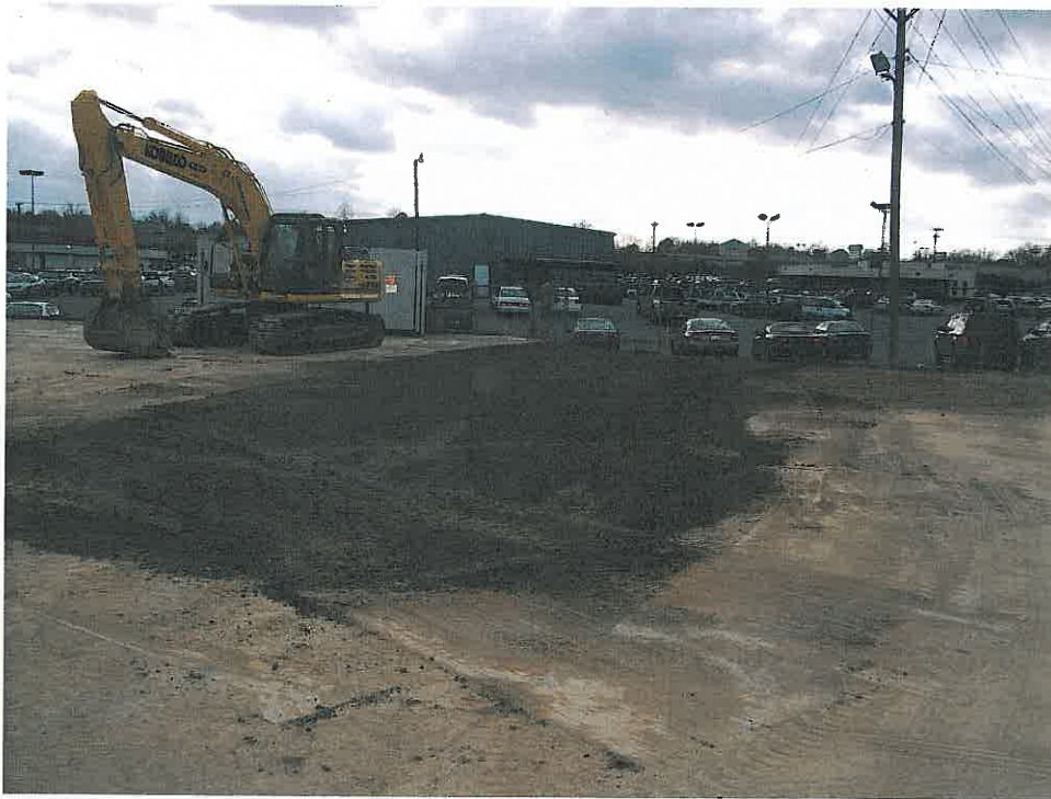
Photograph 12– View of the backfilled excavation.
