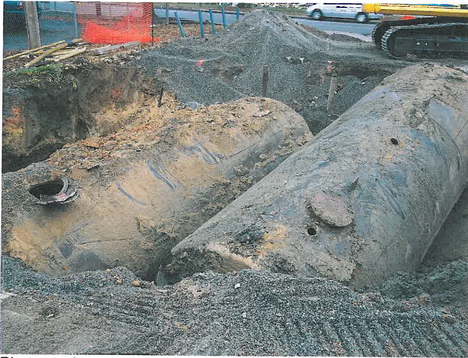
Photograph 7 – View of UST #2 and #3.
