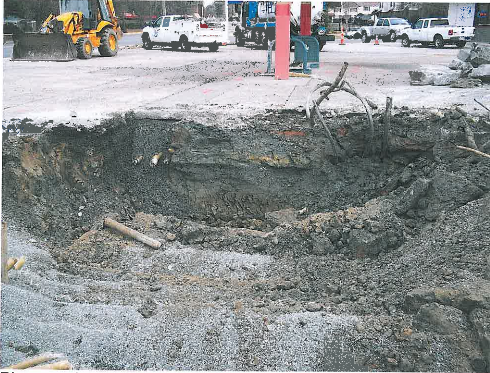
Photograph 9 – View of old and new product piping.
