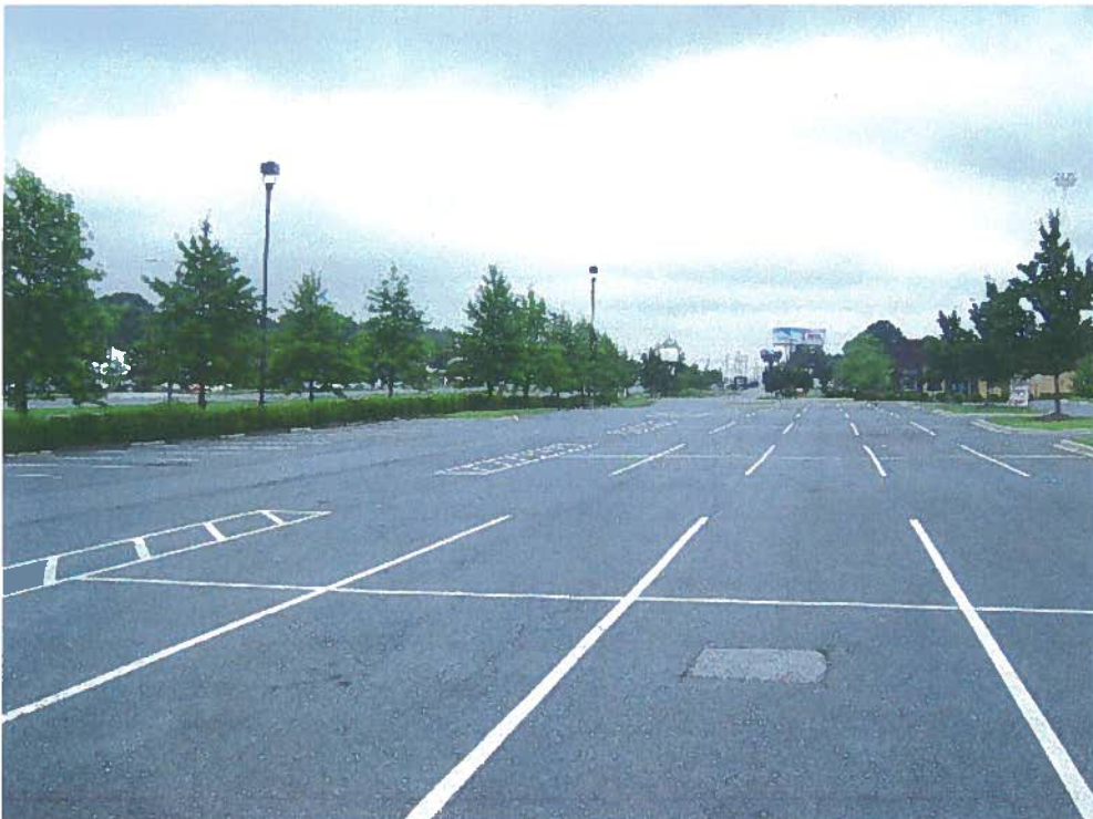
Photograph 2 – View of the southeast side of the BJ's parking lot looking southeast. East Independence Boulevard is shown to the east of the row of trees. Square pavement scar in foreground is the location of an abandoned monitoring well.
