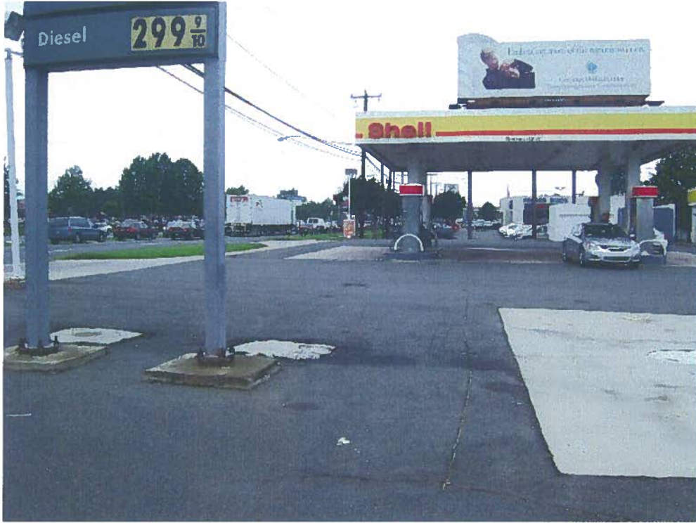
Photograph 3 – View of the western side of the UST field and dispensers of the Shell Sam's Mart property looking north. East Independence Boulevard is shown to the west of the property.
