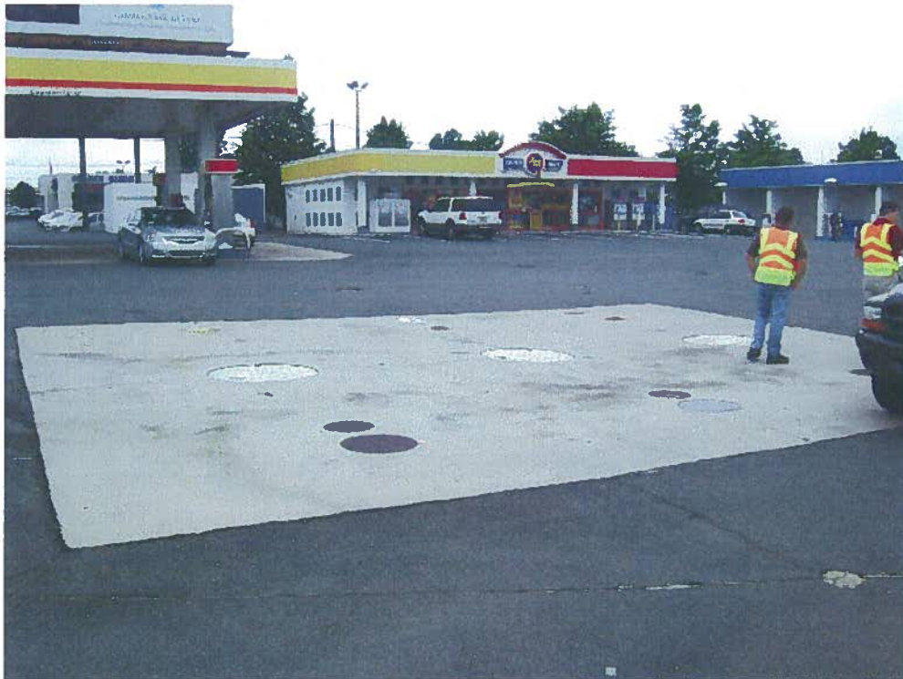
Photograph 2 – View of the UST field of the Shell Sam's Mart property looking north. The dispensers are shown to the west (left) of the store.
