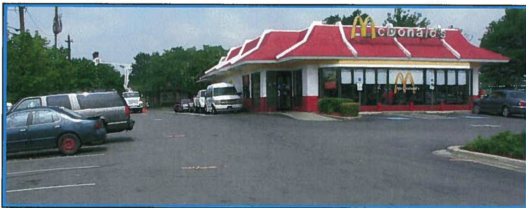
The photograph shows the geophysical survey of the Charlotte Limited Partnership property (Parcel 125) located at the intersection of Independence Boulevard and Idlewild Road in Charlotte, North Carolina. The photograph is viewed in a westerly direction.
