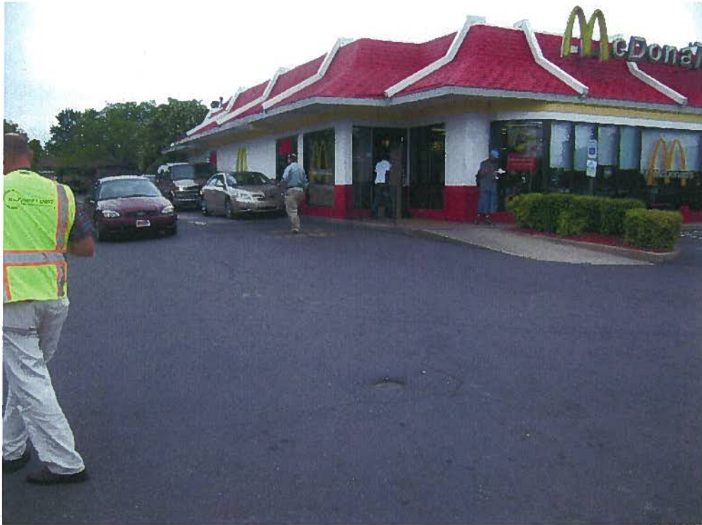
Photograph 1 – View of the McDonald's property looking northwest from the southeastern portion of the property.
