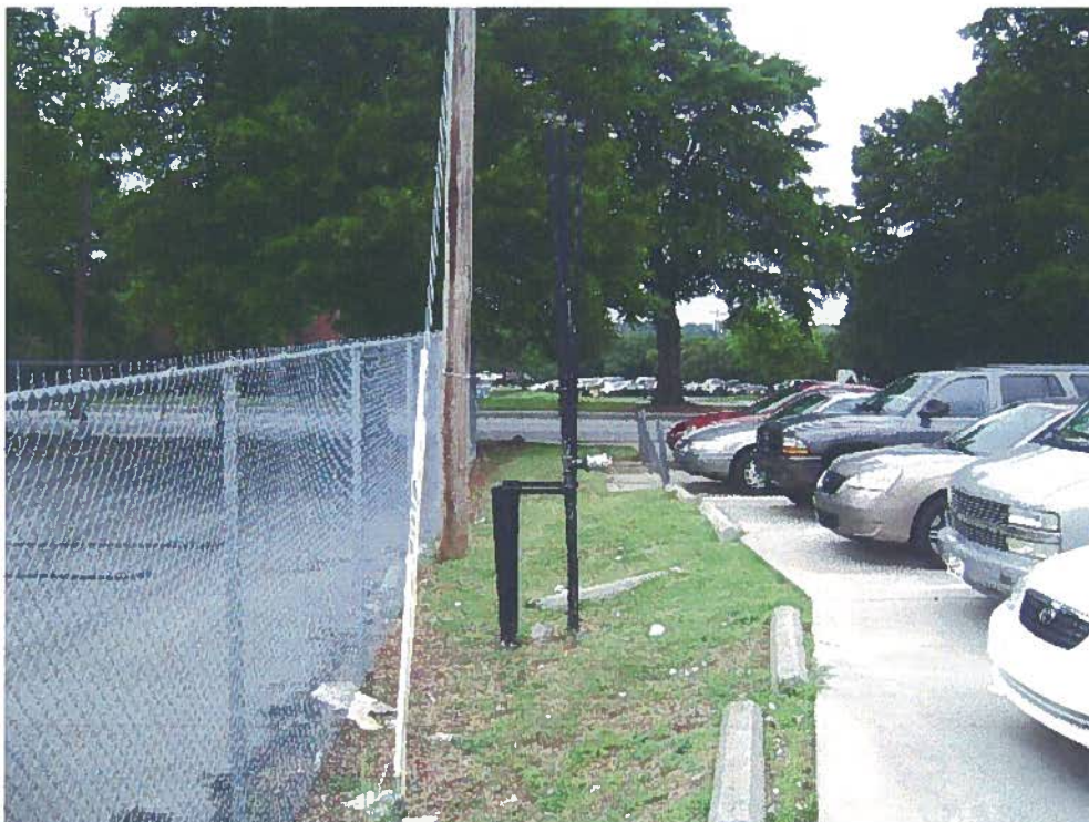
Photograph 4 – View of the west side of the UST field looking north.
