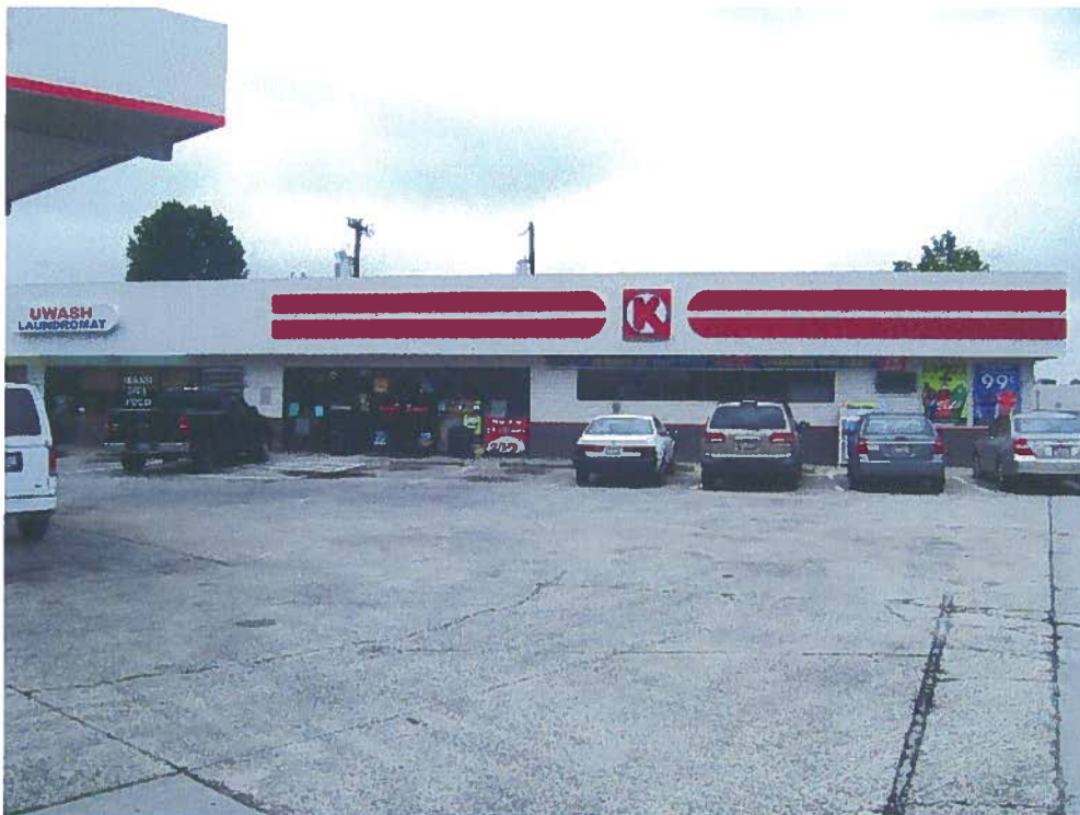
Photograph 3 – View of the southeast corner of UST field in the foreground. Two USTs were closed in 2003 in this area. Refusal encountered at four feet for B-6 in two locations in this area.
