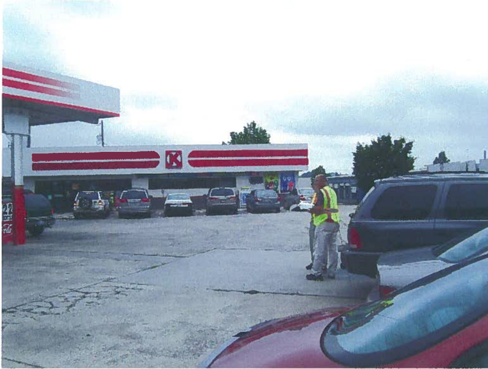
Photograph 1 – View of the Circle K station looking southeast. The UST field is located in the center of the photograph. The dispenser islands are shown to the left (east) of the UST field.
