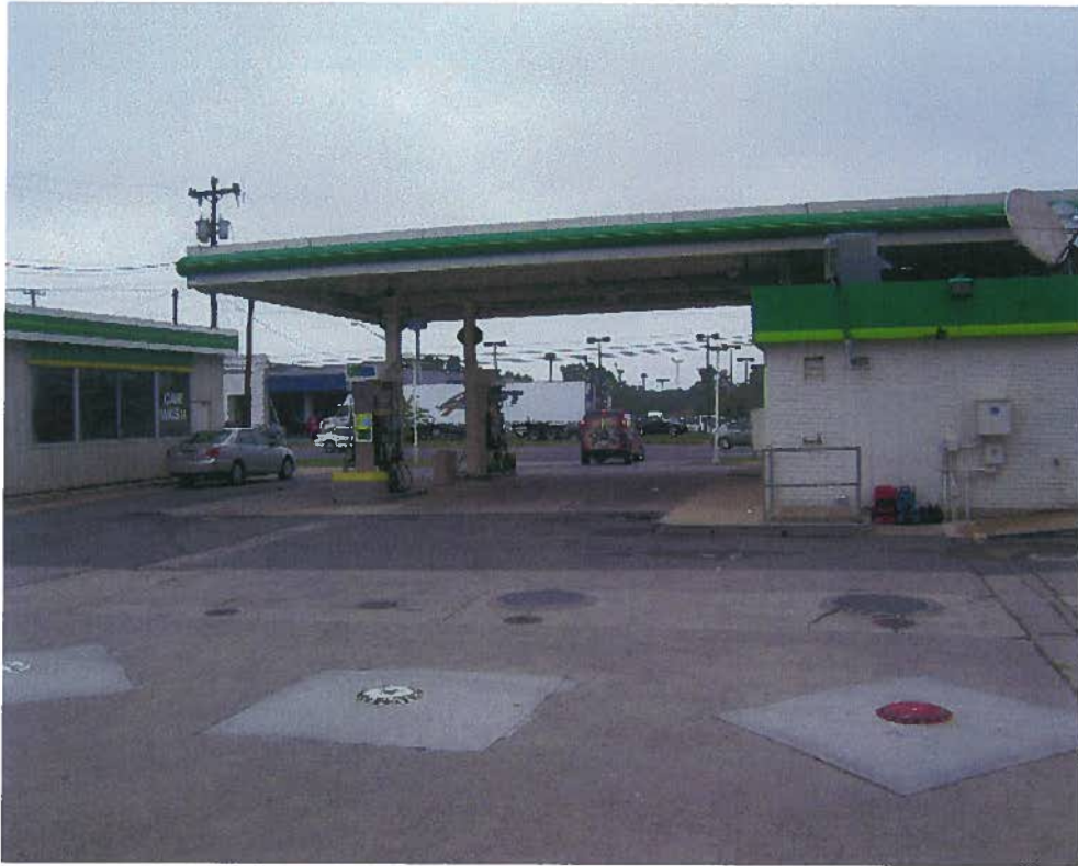
Photograph 1 – View of the Idlewild BP station looking northeast. The UST field is located in the foreground. Two dispenser islands are shown on the north side of the store.
