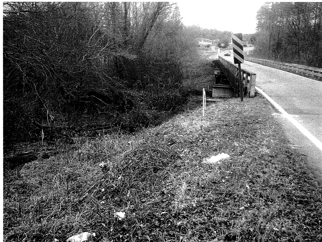
Looking down station from EB2-B
