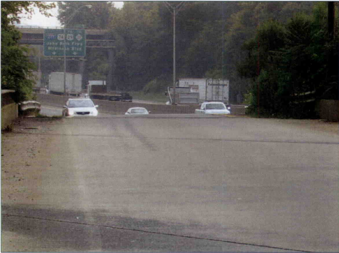
GUARD RAIL LOOKING NORTH
