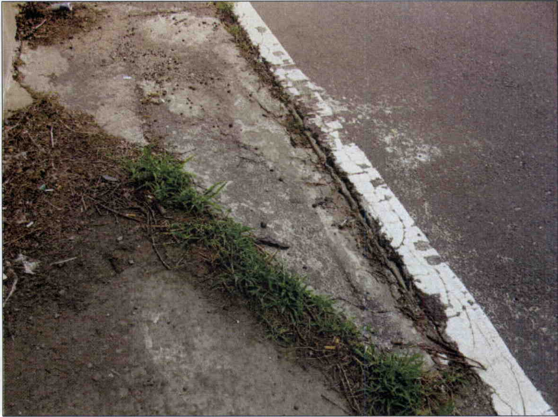
VOID AT THE NE CORNER HAS BEEN REPAIRED WITH GROUT
