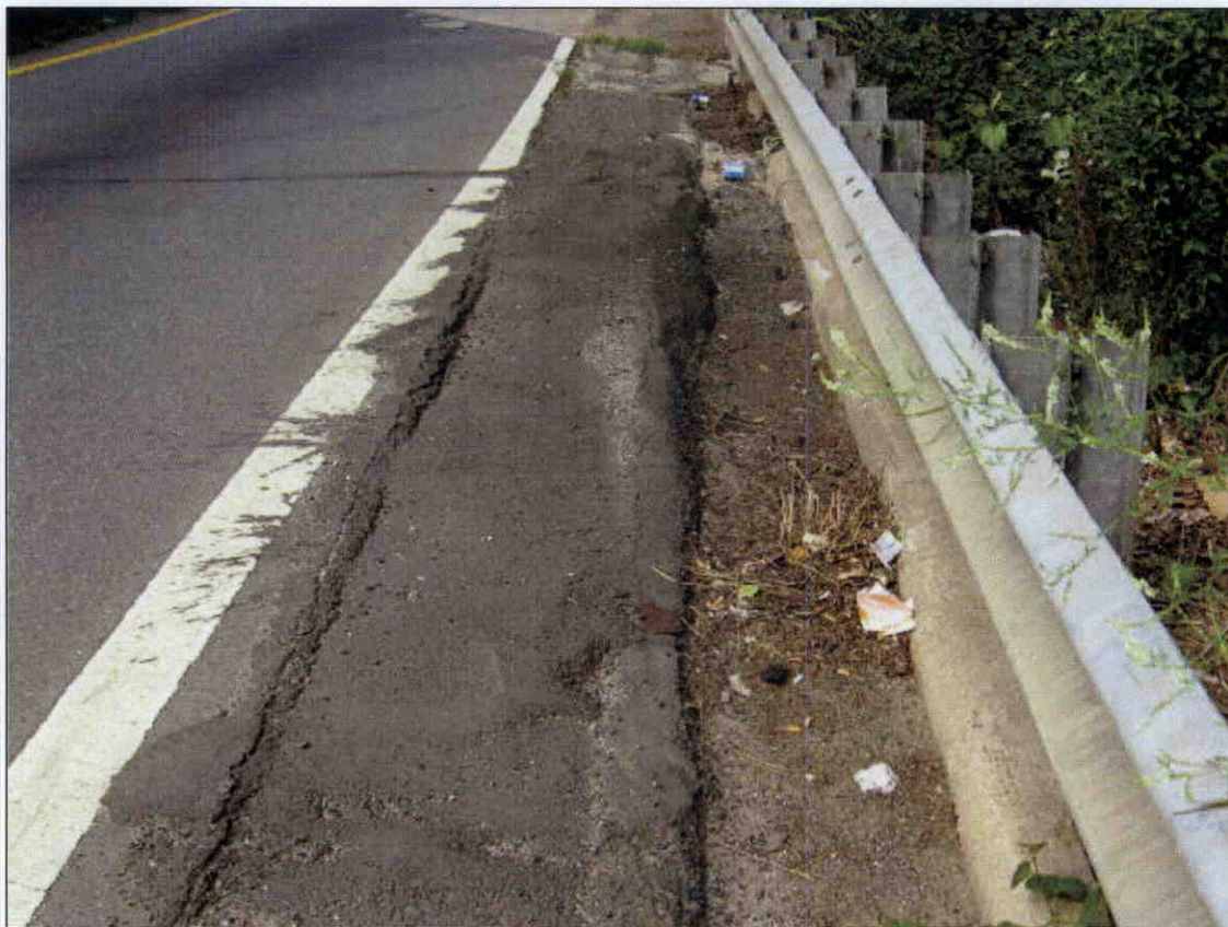
WASH AT NORTH END OF THE BRIDGE LEFT SIDE REPAIRED
