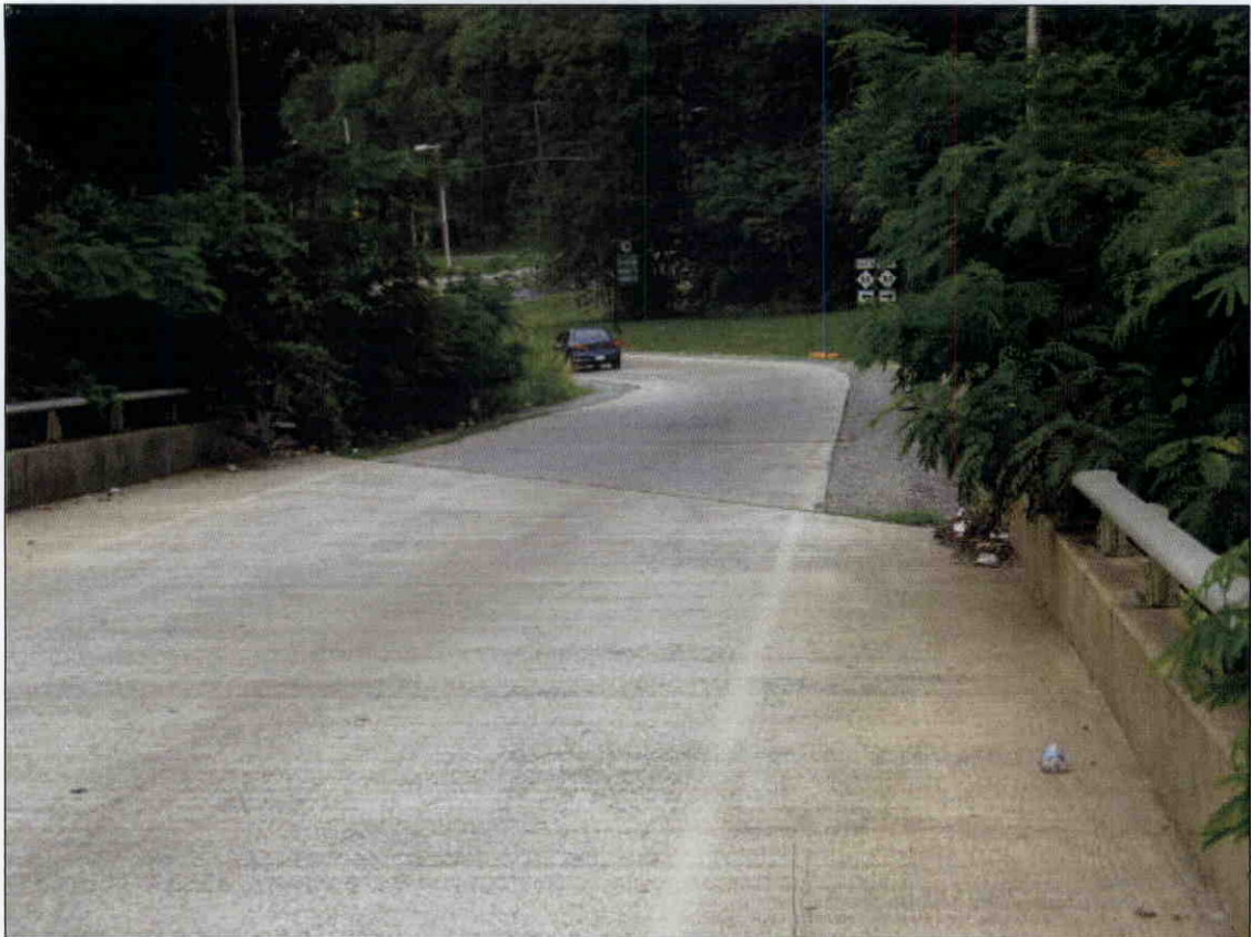
GUARD RAIL LOOKING SOUTH
