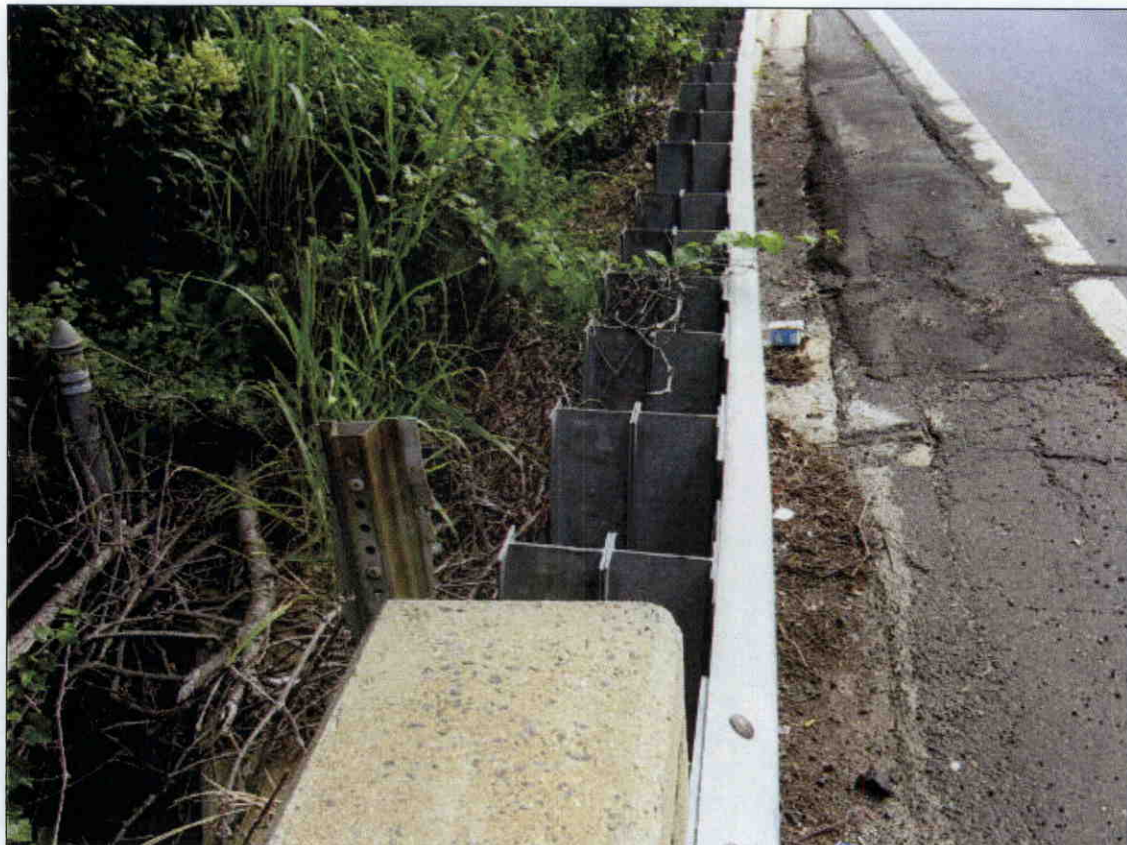
POST SPACING AT THE NW CORNER NE AND SE SIMILAR
