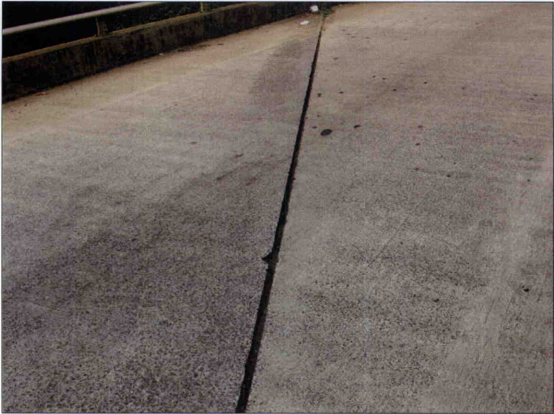
EXPANSION JOINTS AT THE PIERS AND ABUTMENTS
