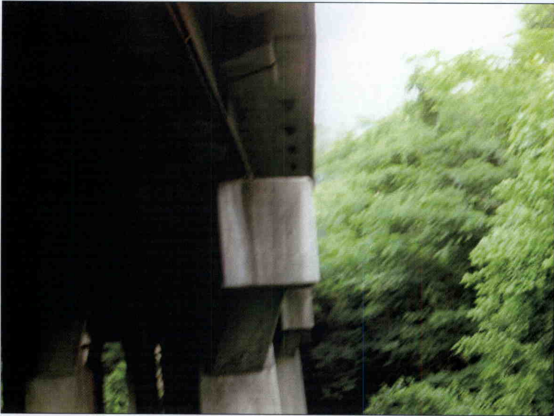
LEFT END OF PIER 3 CAP
