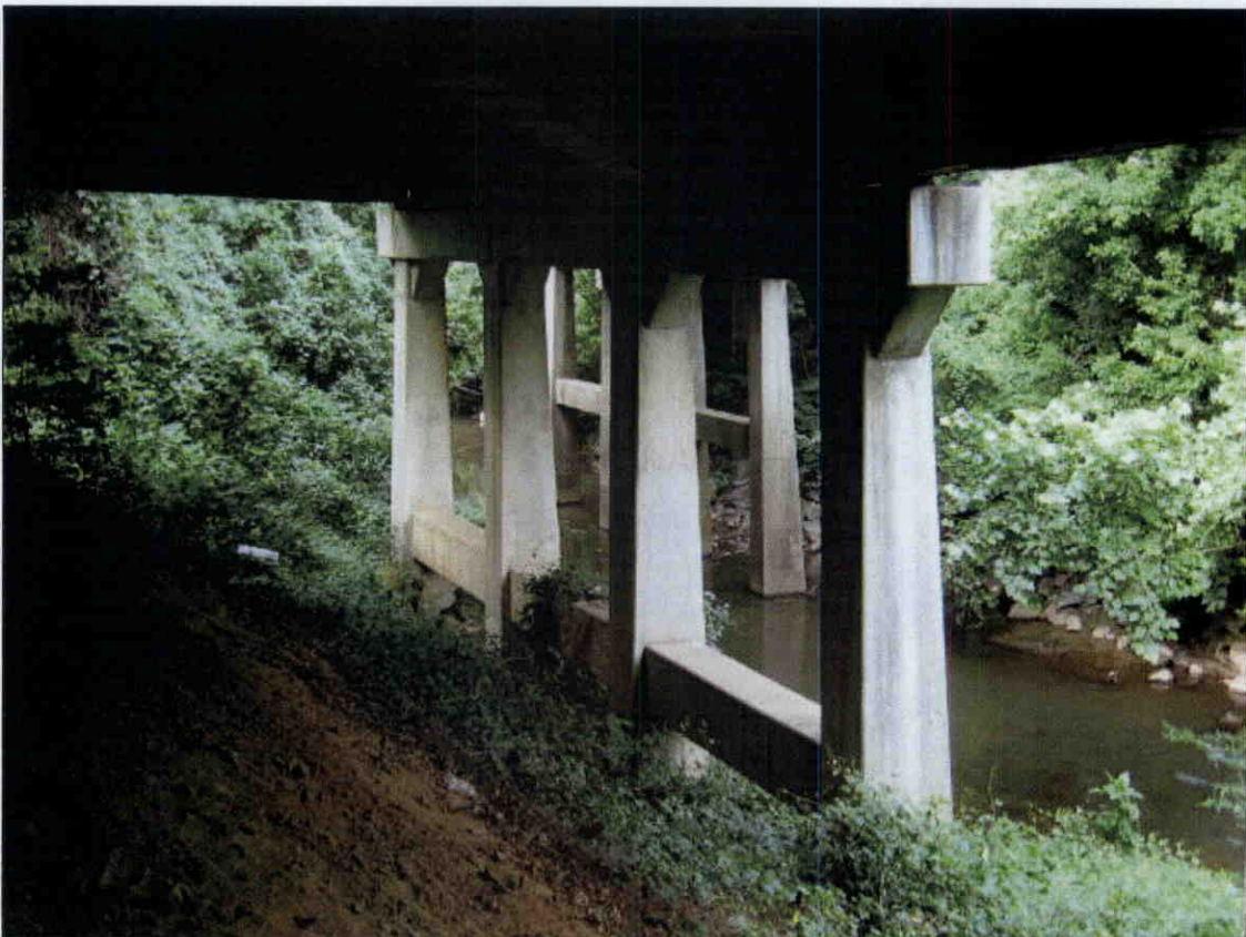
PIER 3 LOOKING SOUTH
