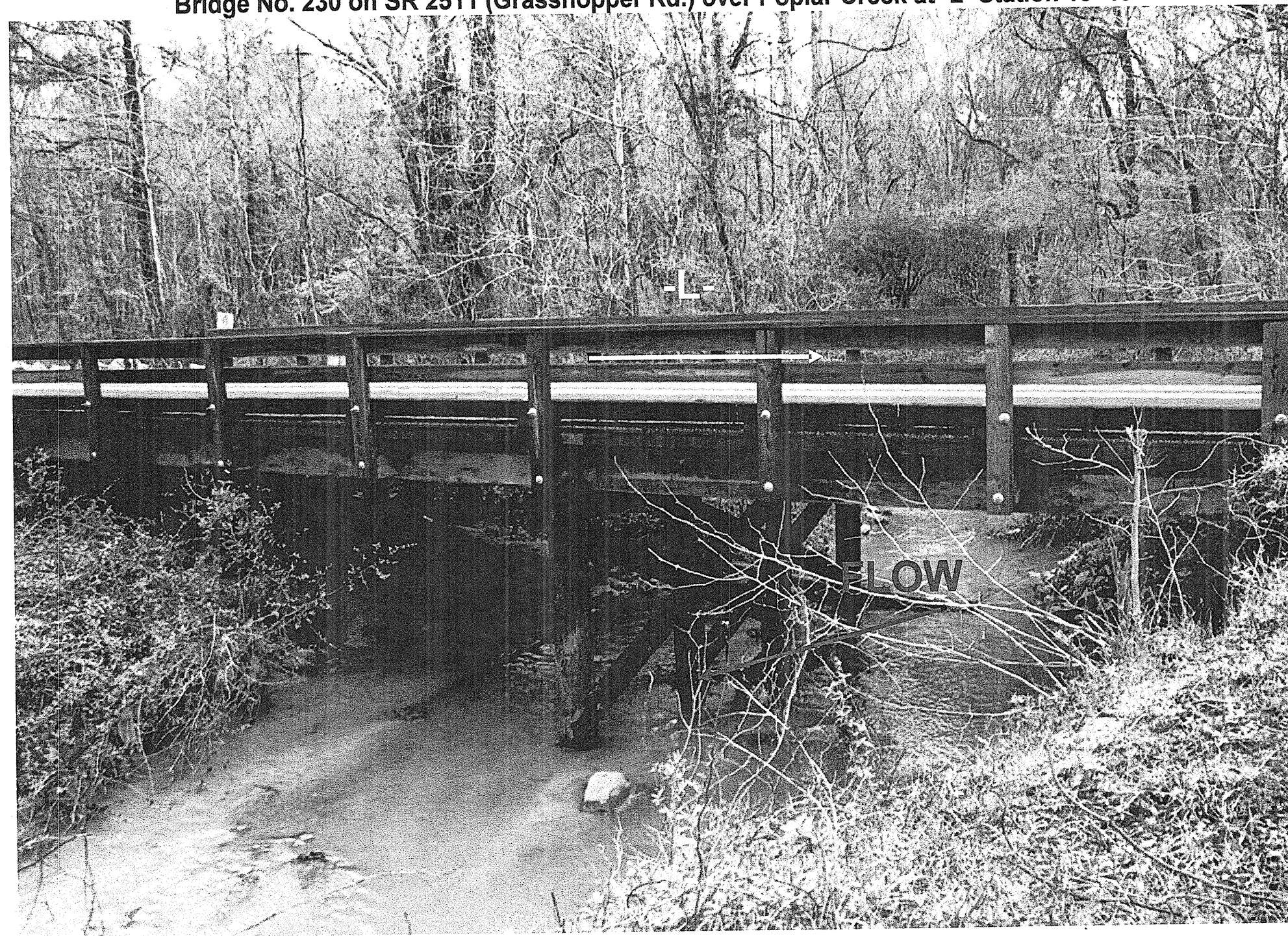
Looking Northwest from End Bent 2
