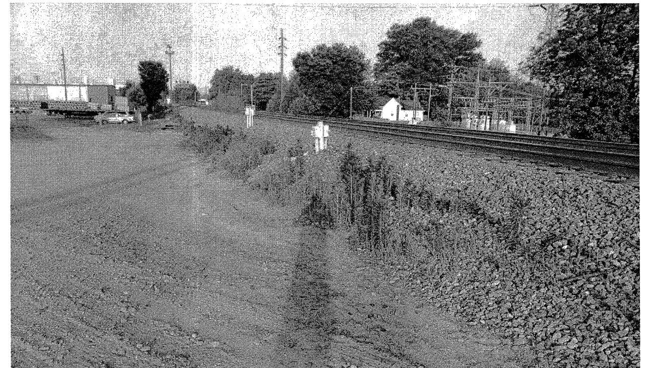
Proposed Bridge Site Looking Southwest
