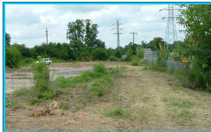
The photo shows the geophysical survey area across the eastern edge of the Former FCX Chemical site located contingent to the Johnson Concrete facility shown above. The photo is veiwed in a northerly direction.
